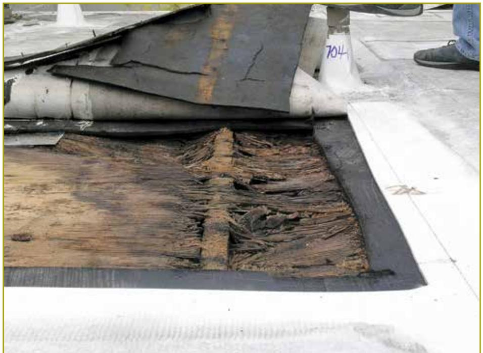
**Figure 1 – Severely deteriorated plywood a few years after replacing an old cap-sheet BUR with a white single-ply roof.**
