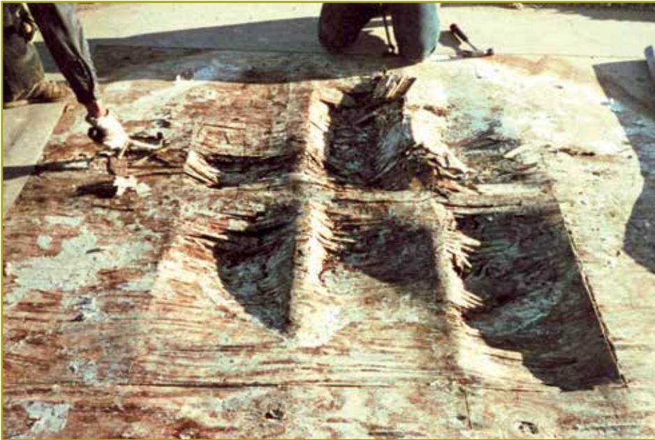
**Figure 2 – Severe deterioration caused by water vapor migrating up through the ceiling of a laundry room.**
