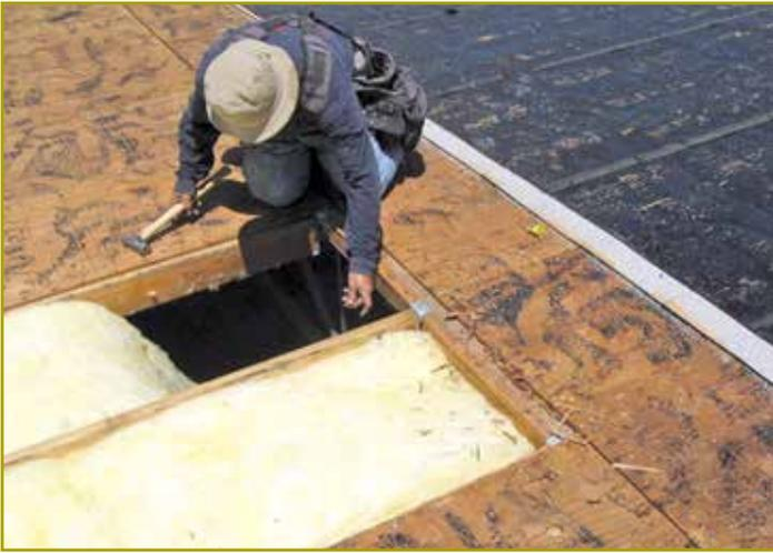
**Figure 7 – Roof construction along truss purlins.**
