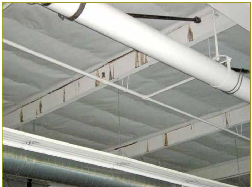
**Figure 3 – Stains on the sides of beams in an office/warehouse building in California.**
