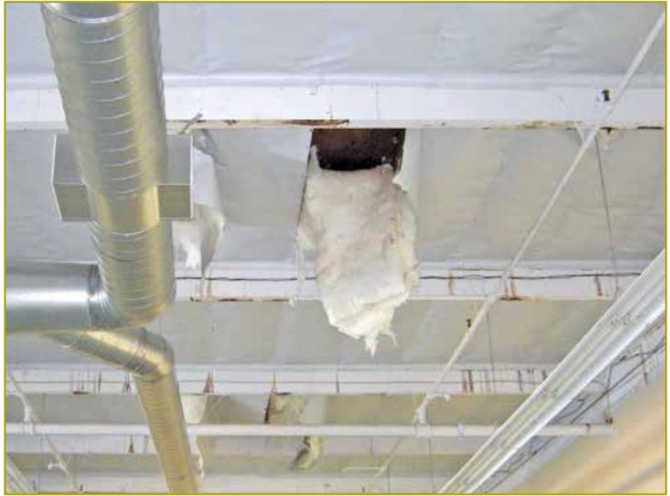
Figure 4 – Water-soaked insulation.
