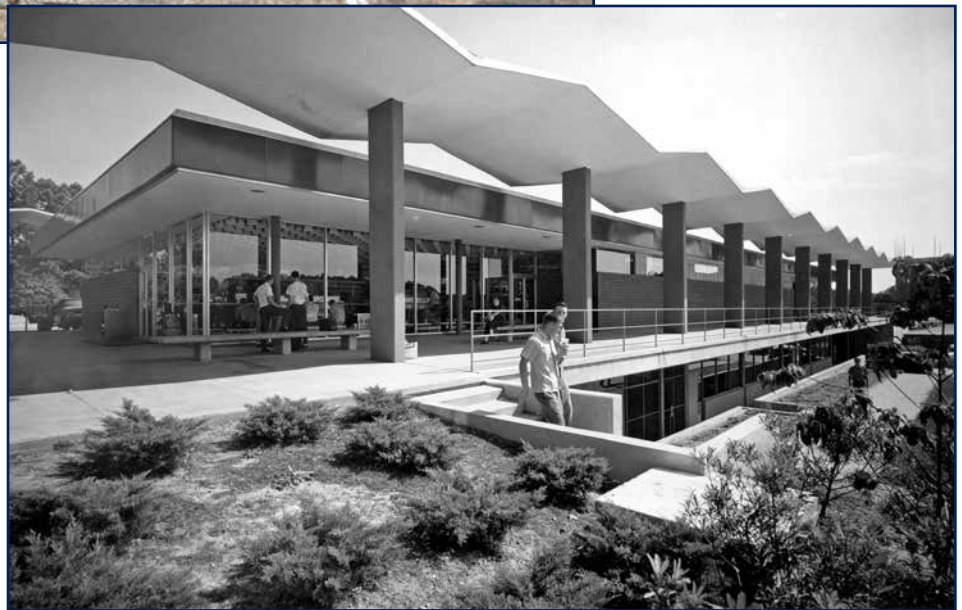
Figure 3 – Folded plate concrete is a less-common variety, relegated more often to older structures.
