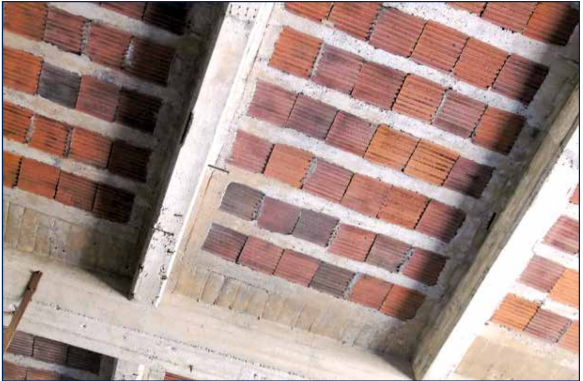
Figure 10 – Concrete roof decks may be poured over structural clay tile (also called “book tile”) situated between concrete beams and columns.
