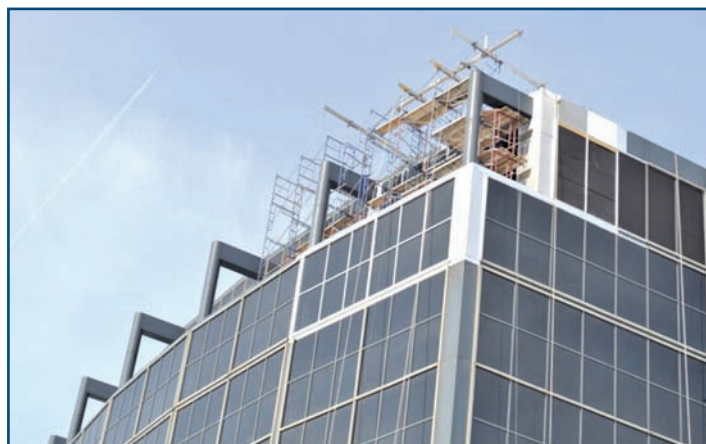
Photo 10 – Pipe scaffolding on setback terraces.
