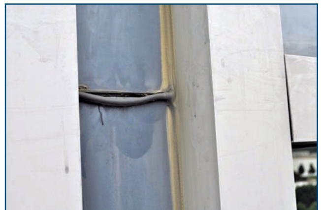
Photo 9 – Failed sealant joint at decorative metal cladding joint.
