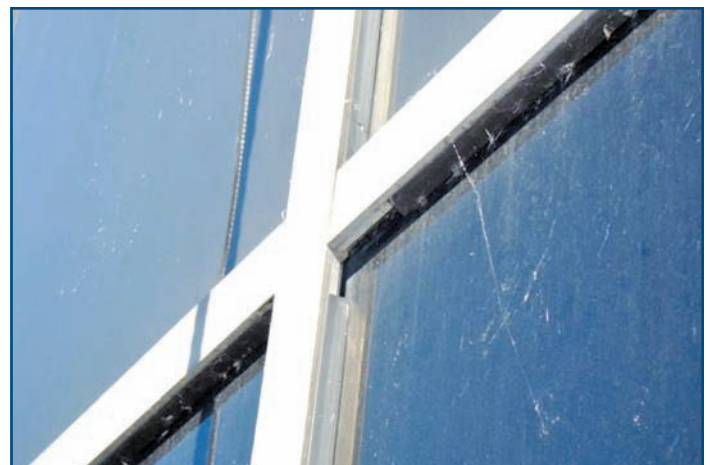
Photo 3 – Extruded glazing gasket shrinkage.
