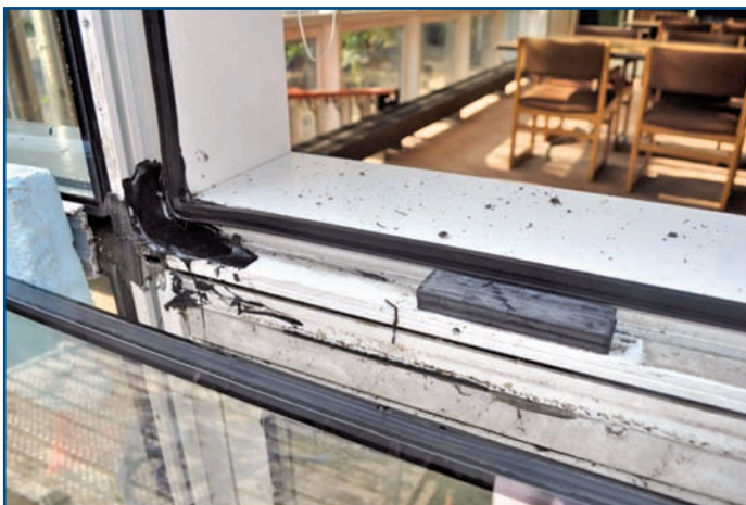
Photo 5 – Repair of internal seals by deglazing.
