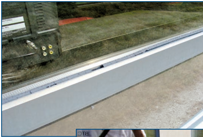
Photo 1 – Crazing of glazing gaskets in a curtain wall system.
