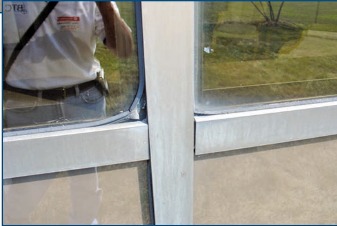
Photo 2 – Shrinkage of glazing gaskets.
