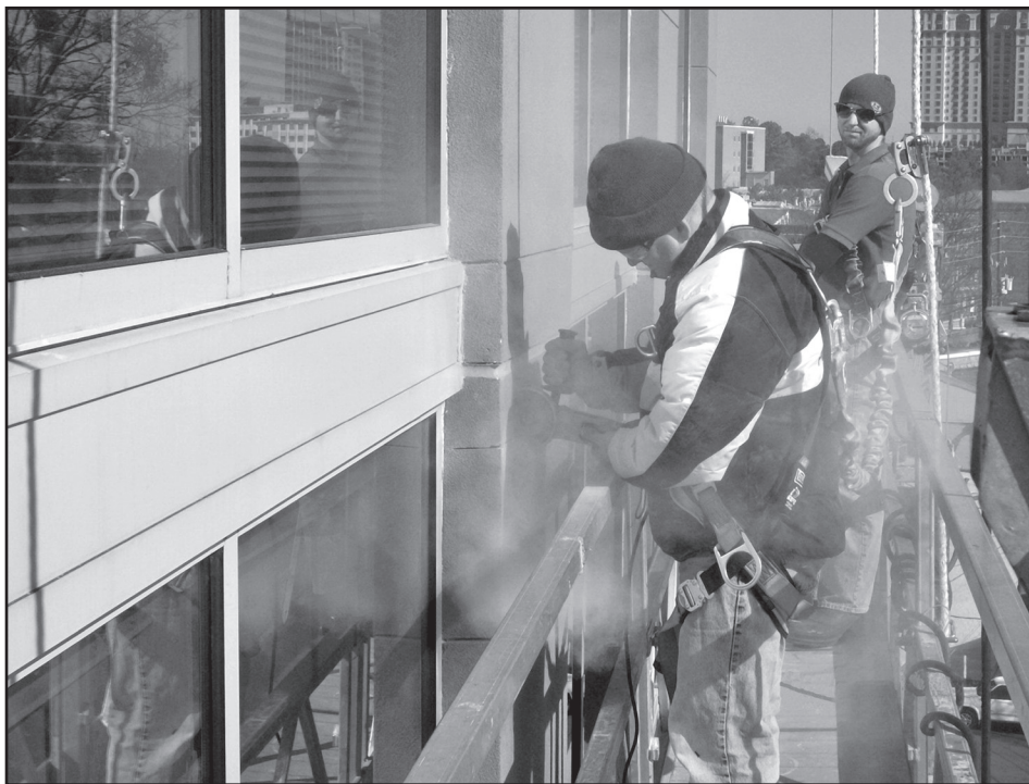
Figure 10 – View of inspection opening in an existing stucco high-rise wall assembly to evaluate effectiveness of the proposed repair.
