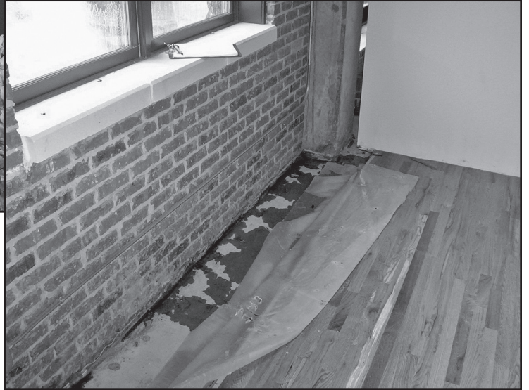
Figure 3 – View of significant water infiltration and deteriorated interior finishes.
