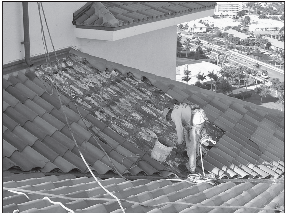
Figure 1 – View of a large inspection opening on a steep clay-tile roof of a high-rise condominium.
