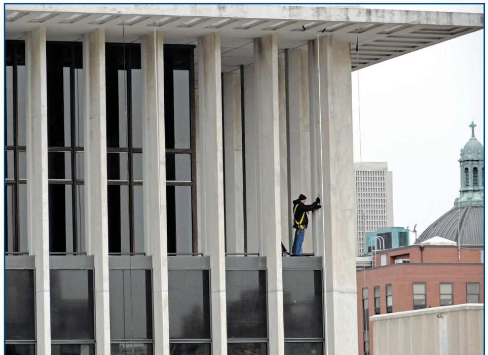
Figure 4 – Marble fin panels continuing past the ninth-floor terrace.
