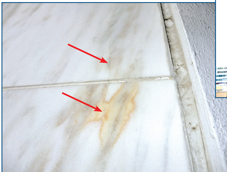
Figure 7 – Vertical crack approximately 4-5 inches in length, emanating from the intermediate marble panel joint at the ninth-floor marble fin panel.
