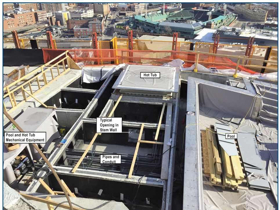
Figure 1 – Pool and hot tub installation in progress.
