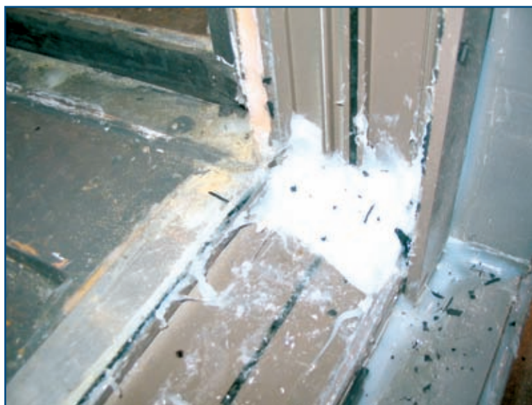
Photo 6 – Extremely heavy corner seal.
