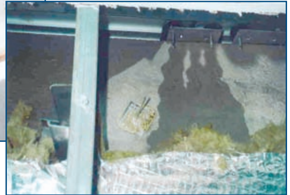
Photo 8 – Heavy leakage is shown through a splice in the sub-sill (shown in Photo 7) due to failed seal with irregularly spliced material (viewed from interior and below, with interior finishes and insulation removed to expose the leakage).
