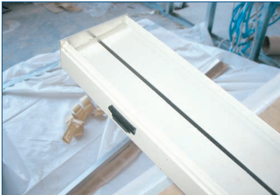
Photo 1 – Sample sub-sill with sealed end dam installed. Also note the black weep cover (which covers a slotted weep hole) and the slope to the exterior.
