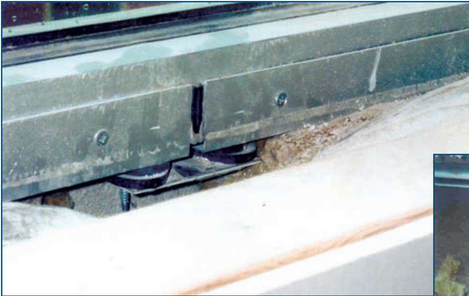
Photo 7 – Up-close view of a splice joint in a sub-sill (viewed from interior, with interior finishes removed). Note the corrugated profile of the splice material.
