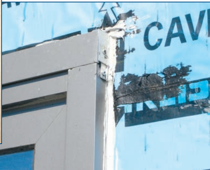
Photo 5 – Large end cap installed at ends of the head receptor.
