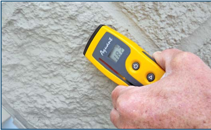
Photo 7 – Instrument used on CMU with coating.
