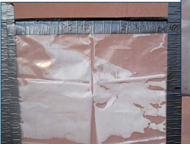
Photo 3 – Plastic sheet test in place overnight.
