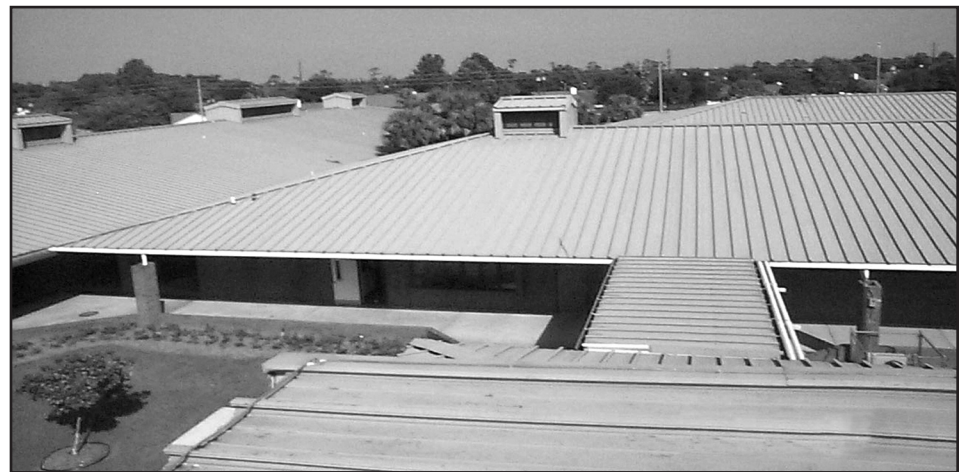
Photo 11 – The school's existing condition shows the dead-level valley with the internal gutter and several ventilation cupolas.
