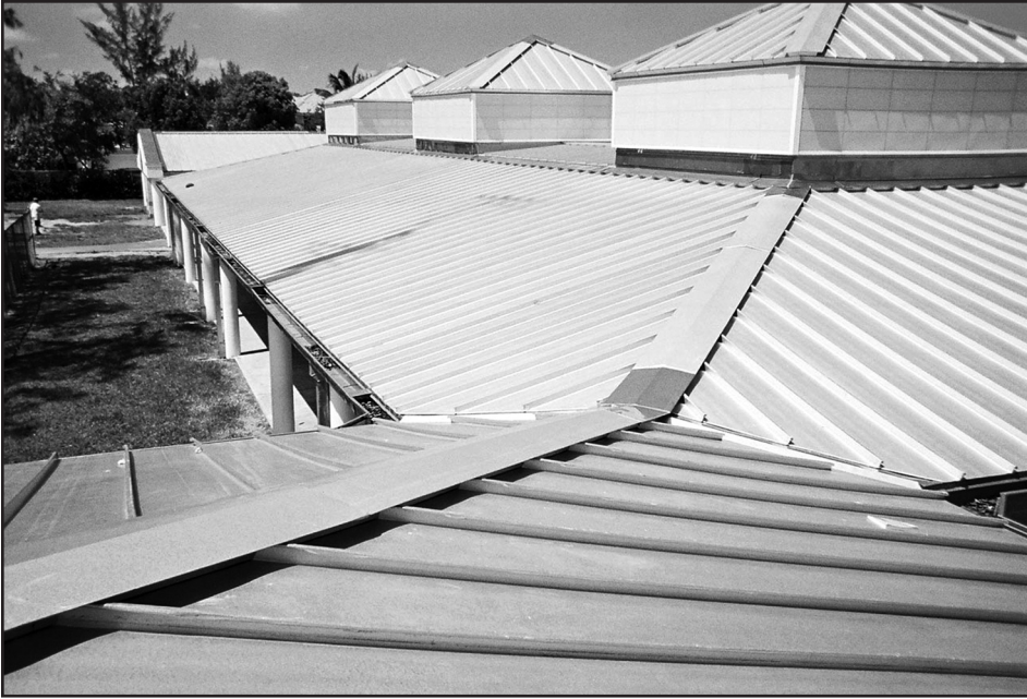
Photo 4 – New roof at Broward County school.
