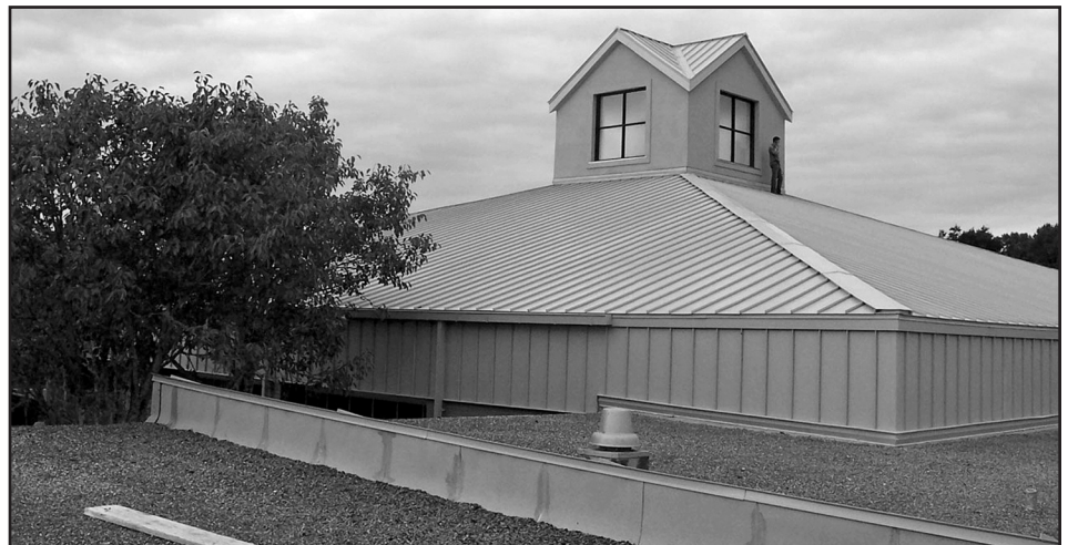
Photo 15 – A portion of the media center's refurbished roof.
