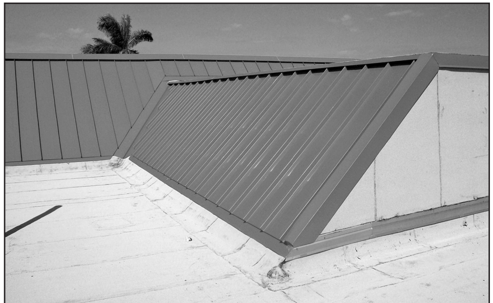
Photo 5 – Roof at Imperial Point Library.
