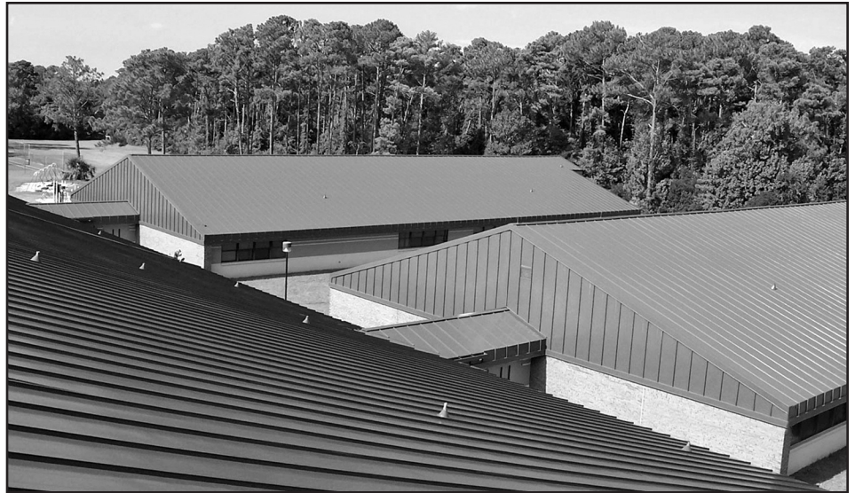
Photo 16 – Portion of completed roof.
