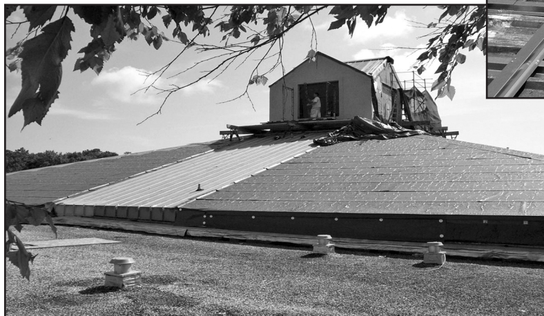
Photo 1 – Replacement of an architectural roof panel over a solid substrate.
