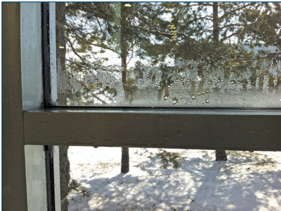
Figure 2 – Surface condensation on glass.
