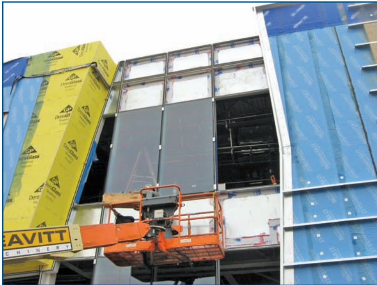
Figure 22 – Using membrane to create vapor seal at nonwelded joints.
