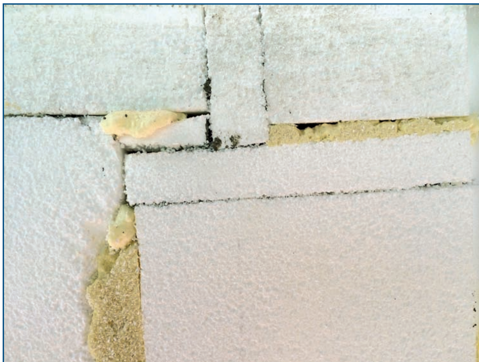
Figure 13 – Filling large gaps with SPF in EIFS assembly.
