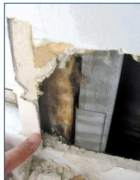
Figure 8 – Mold due to interstitial condensation.
