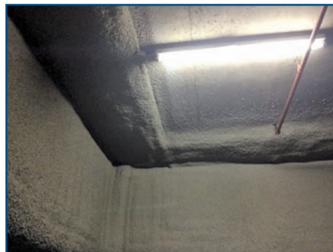
Figure 26 – Insulated parking garage slab.
