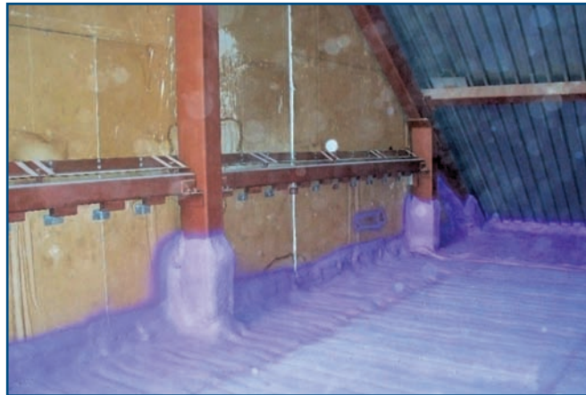
Figure 35 – Foam insulation as prime barrier in attic.
