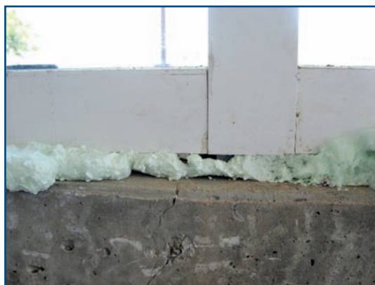
Figure 16 – Low-expansion foam insulation.
