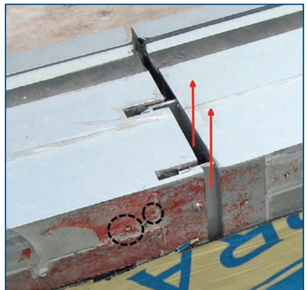
Figure 30 – Air leakage through mullions.
