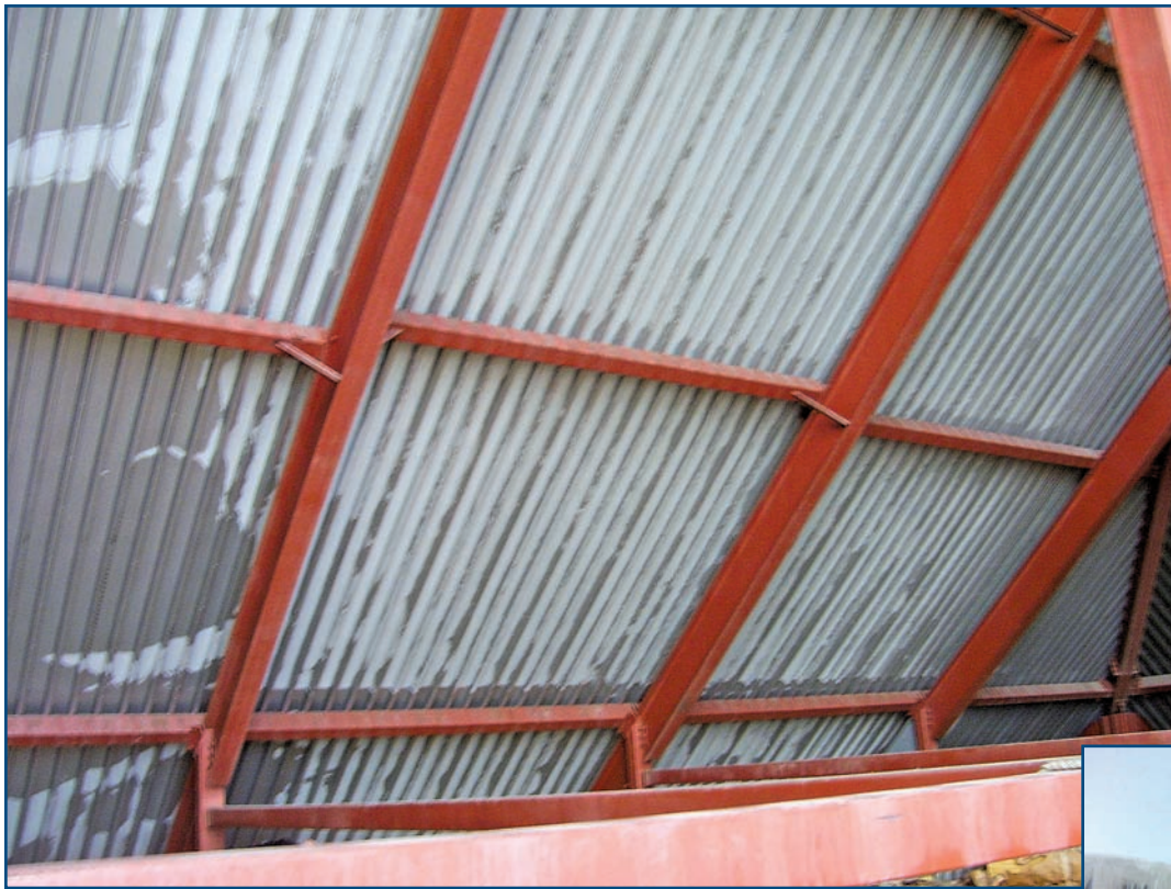
Figure 33 – Condensation and frost on the attic wall.
