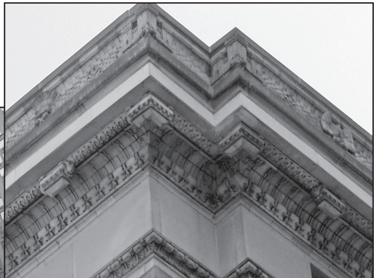
Photo 2 – Ornate terra cotta cornice and parapet wall.
