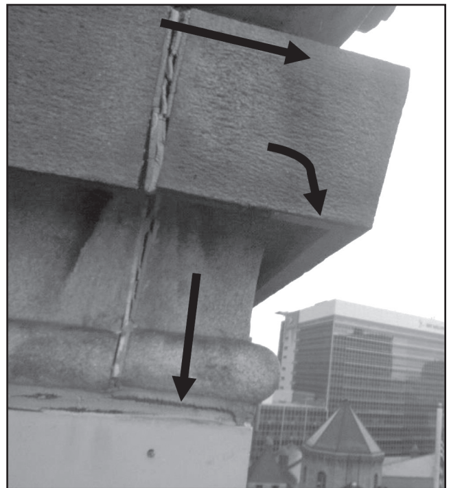
Photo 6 – Granite water table at the corner of the cornice was noted to be rotating down and out from the corner
