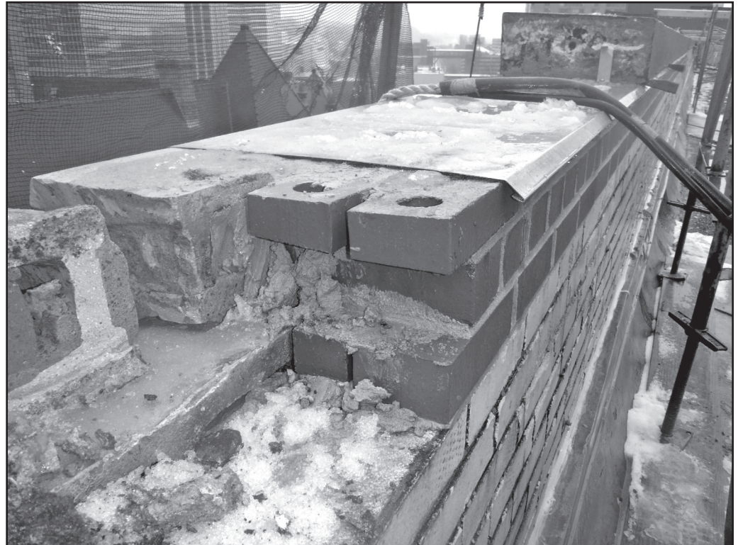
Photo 8 – Limited rebuild of masonry parapet wall and installation of metal through-wall flashing. Note half brick (approximately 2 in. high) used at top of wall; this represents the amount of swell in the remainder of the wall due to irreversible expansion of the masonry.
