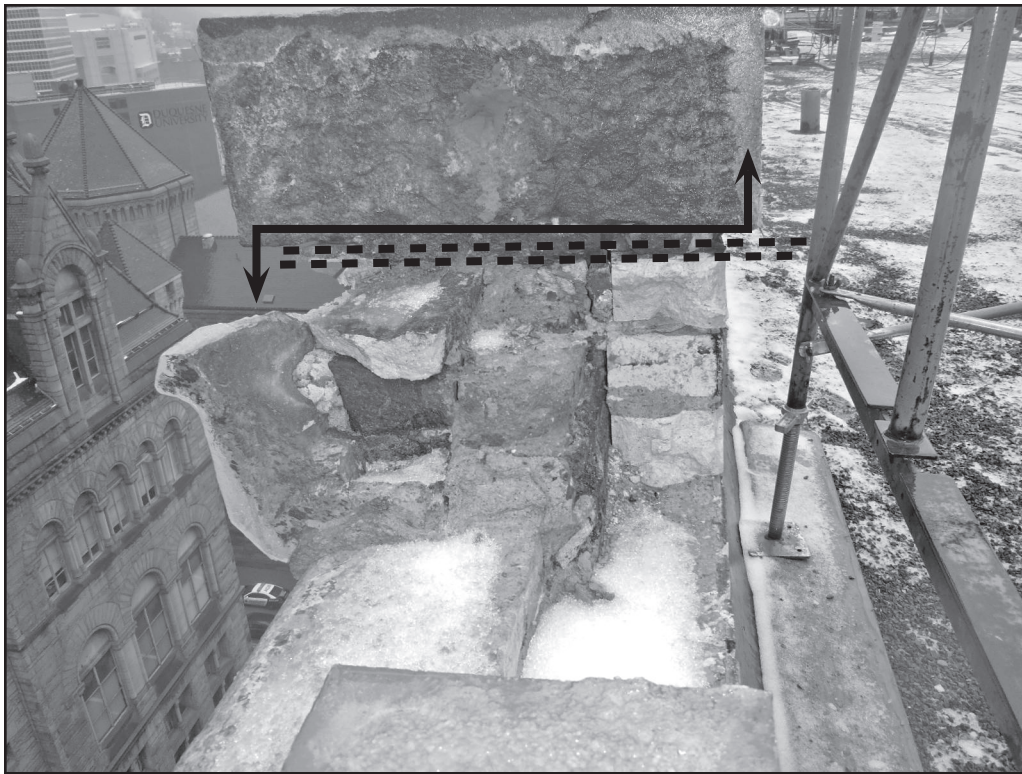
Photo 4 – Cross-section of parapet coping. Arrows indicate rotation of coping. Solid line is approximately level to show amount of rotation. Dashed lines indicate differential amount of heave in back-up masonry due to irreversible moisture expansion.
