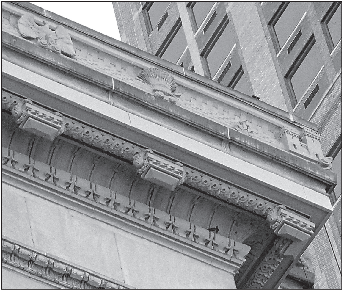
Photo 10 – Completed repairs at terra cotta cornice and parapet.
