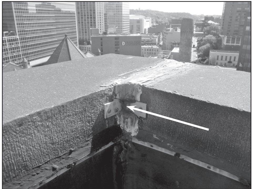
Photo 3 – Thermal and moisture expansion within the brick and granite parapet wall elements caused a pushing motion to occur at the corners of the perimeter wall.
