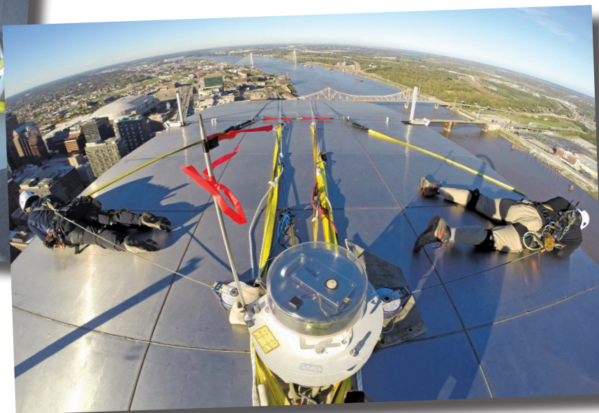
Figure 5 – Custom IRA system at the top of the Gateway Arch.
