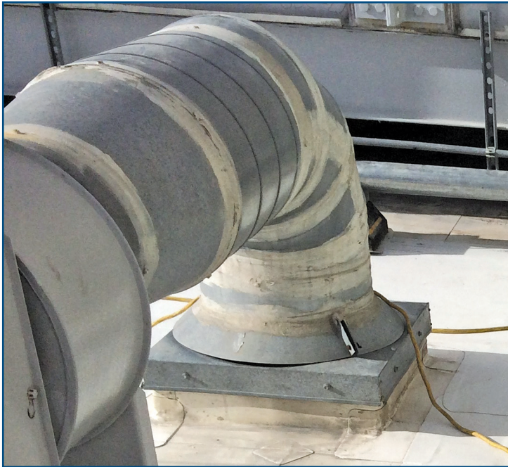
Figure 6 – Typical duct penetration.
