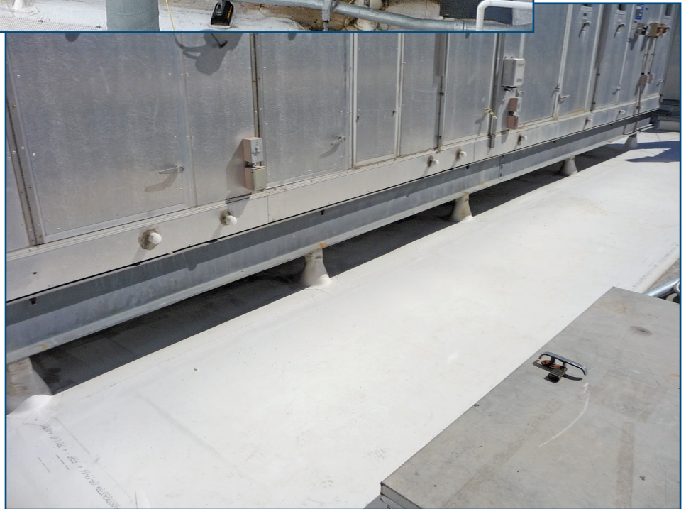
Figure 5 – Close-up of unit mounted on posts.
