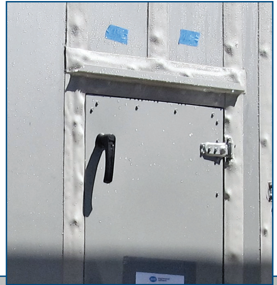
Figure 8 – Preformed silicone tape over all joints in AHU.
