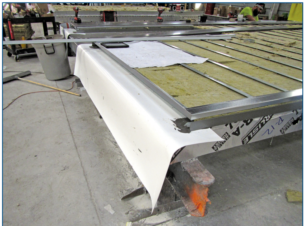
Figure 8 – Roof membrane transition to prefabricated panel.
