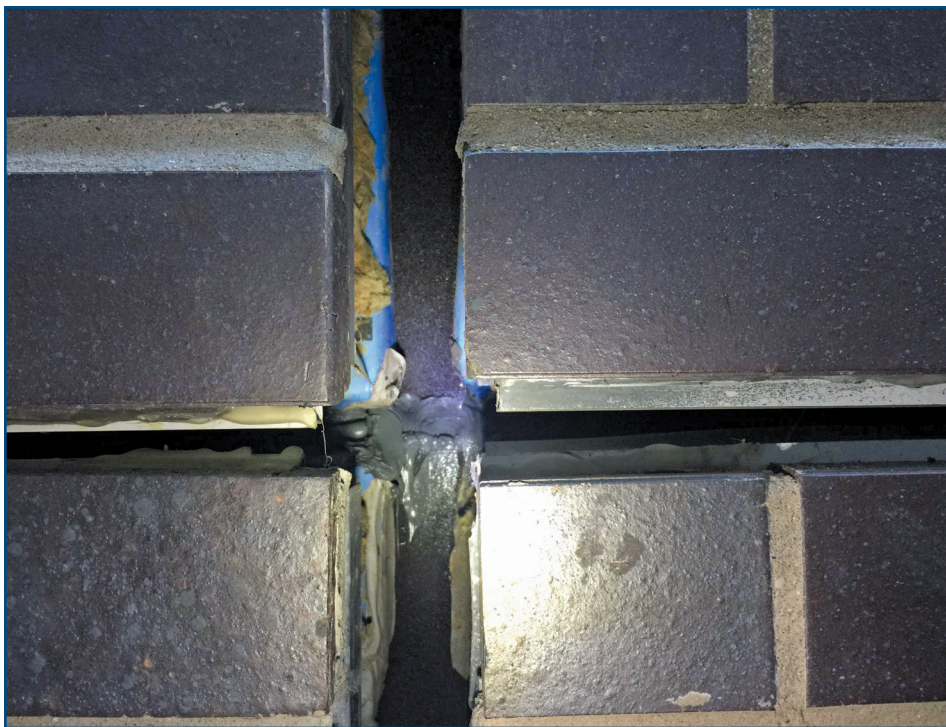
Figure 5 – Expandable foam tape with sealant at the panel corner.
