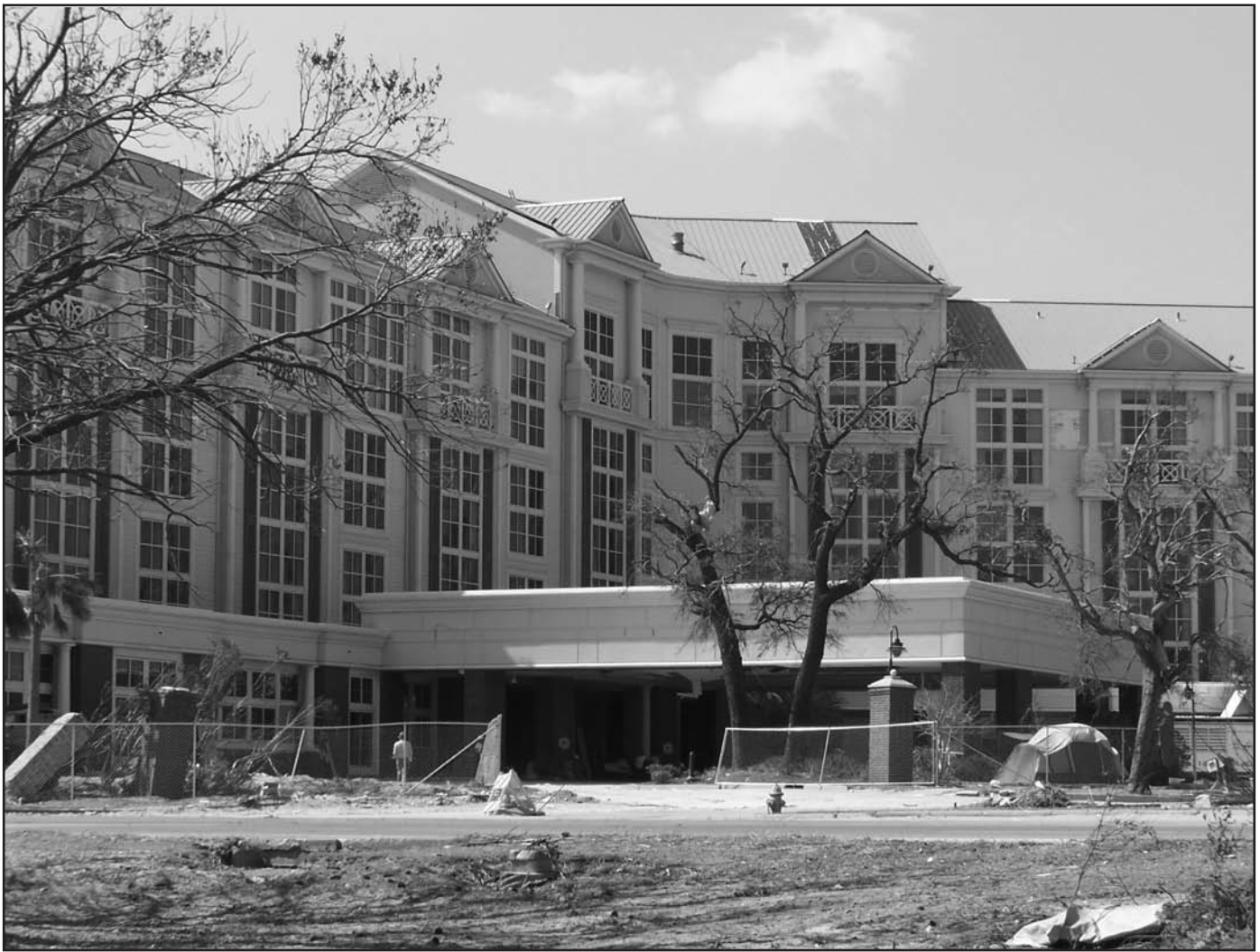
Figure 2 – Characteristic successful performance of code-compliant glazing (wind pressure-rated and impact-resistant) on Island View Casino Resort, Gulfport, MS, during Hurricane Katrina (photo by M. Fischer).
