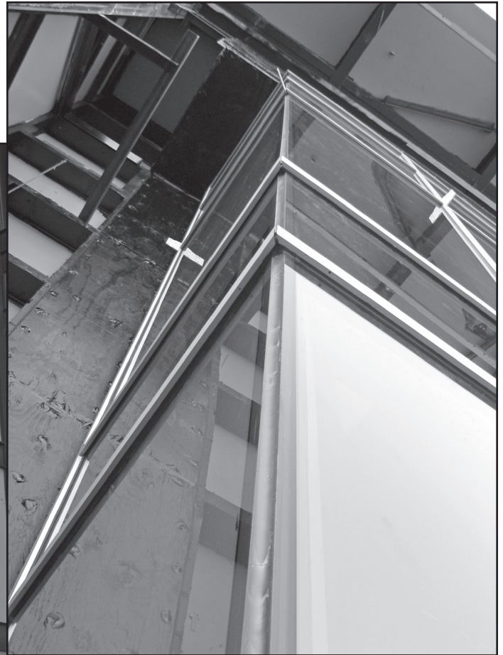
Figure 4 – Outside corner of unitized curtain wall mock-up.
