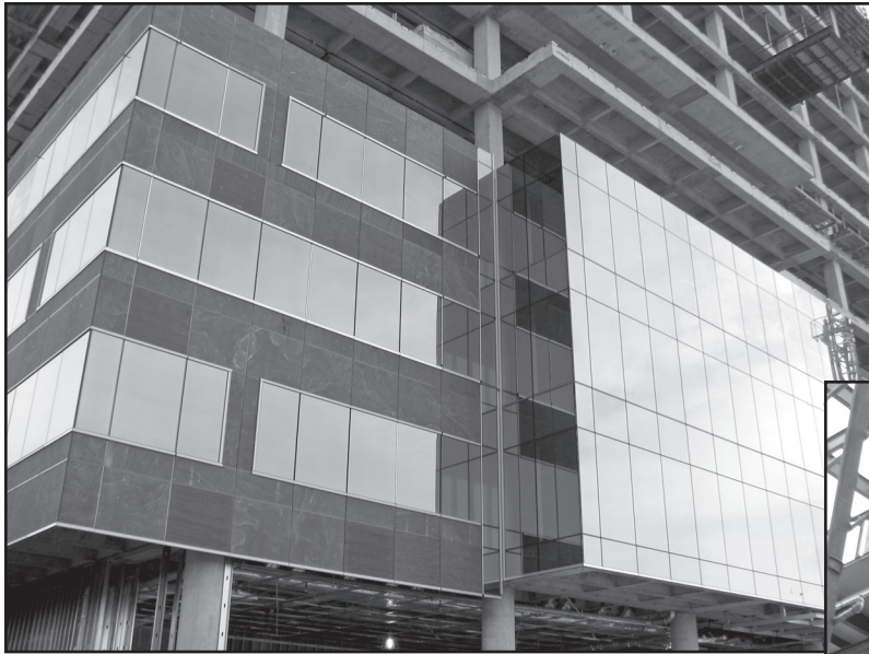
Figure 16 – Case Study #2—a 12-story commercial office building.
