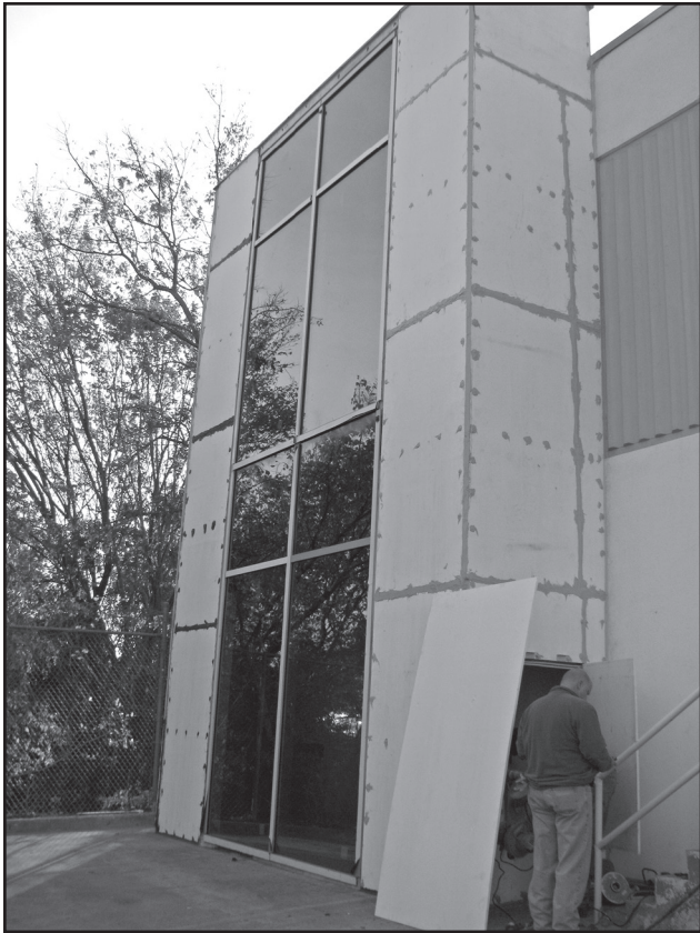
Figure 13 – Two-story unitized mock-up of typical floor spans.
