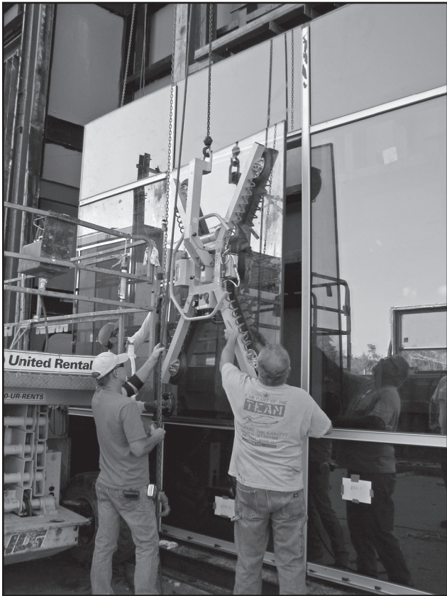
Figure 6 – Reglazing of unitized mock-up.
