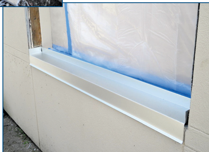
Figure 15 – New custom-built sill pan with integrated end dams.
