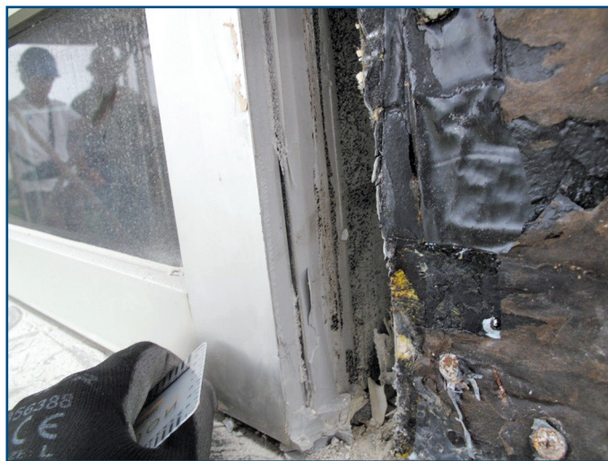
Figure 9 – Large gap at curtainwall jamb and no WRB or flashing wrapped in rough opening.
