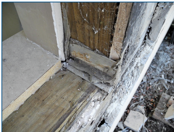
Figure 14 – End dams directly connected to rough opening rather than sill pan. Note the WRB terminating at vertical face of sheathing and not wrapped into rough opening.
