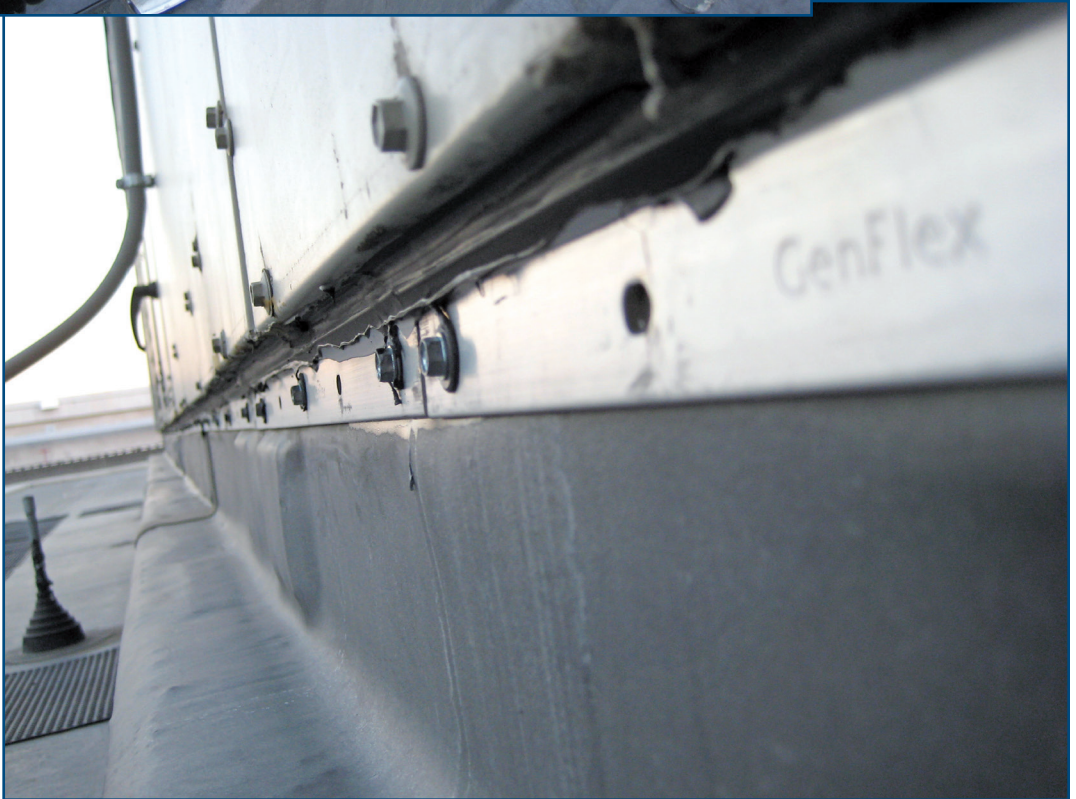
Figure 11 - Roof membrane terminated to base of wall panel.
