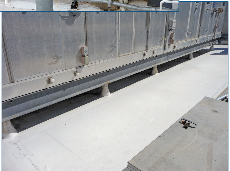
Figure 5 – Close-up of unit mounted on posts.
