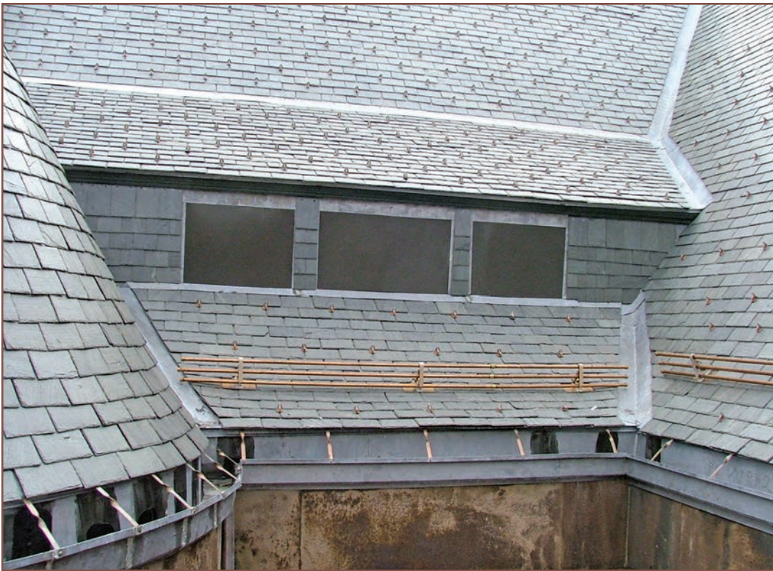
Figure 6 – Snow guard installation.
