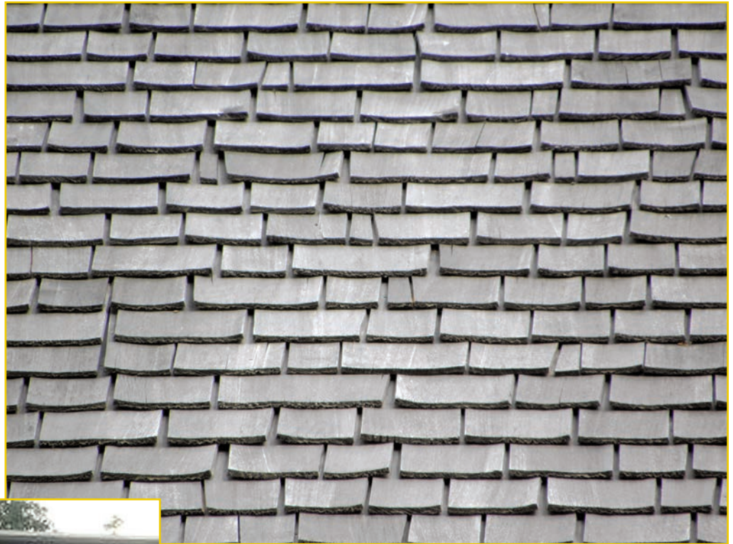
Photo 3 – Nonpermeable membrane used beneath shingles across entire roofing deck.
