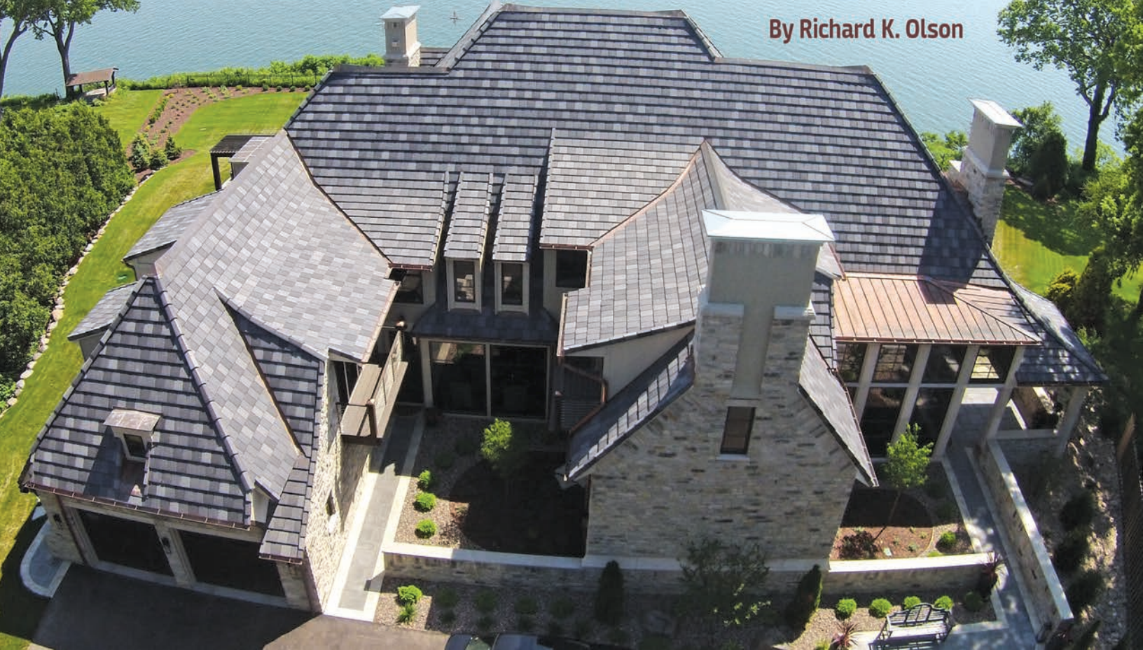
Figure 1 – Concrete flat-tile installation.
