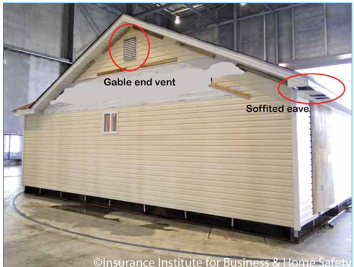
Figure 1 – End view of the building, showing location of gable end vent (open) and soffited eave. Note: Some of the panels have detached as a result of exposure to the elevated wind speeds.
