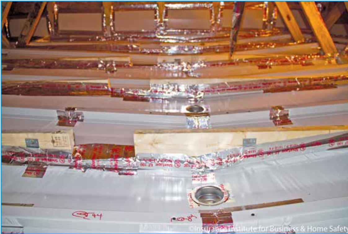
Figure 2 – Water collection channels between ceiling trusses in the attic of the test building.
