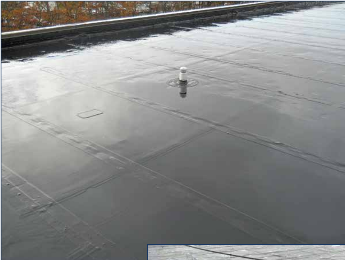
Figure 6 – Disbonded EPDM membrane area in foreground; adjacent area in background is still bonded.
