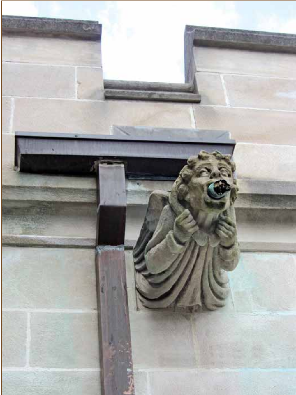
Photo 2 – Original scupper drain with 2000 retrofit gutter.
