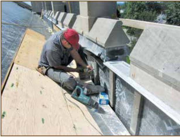
Photo 9 – Nave parapet wall vent construction in 2012.
