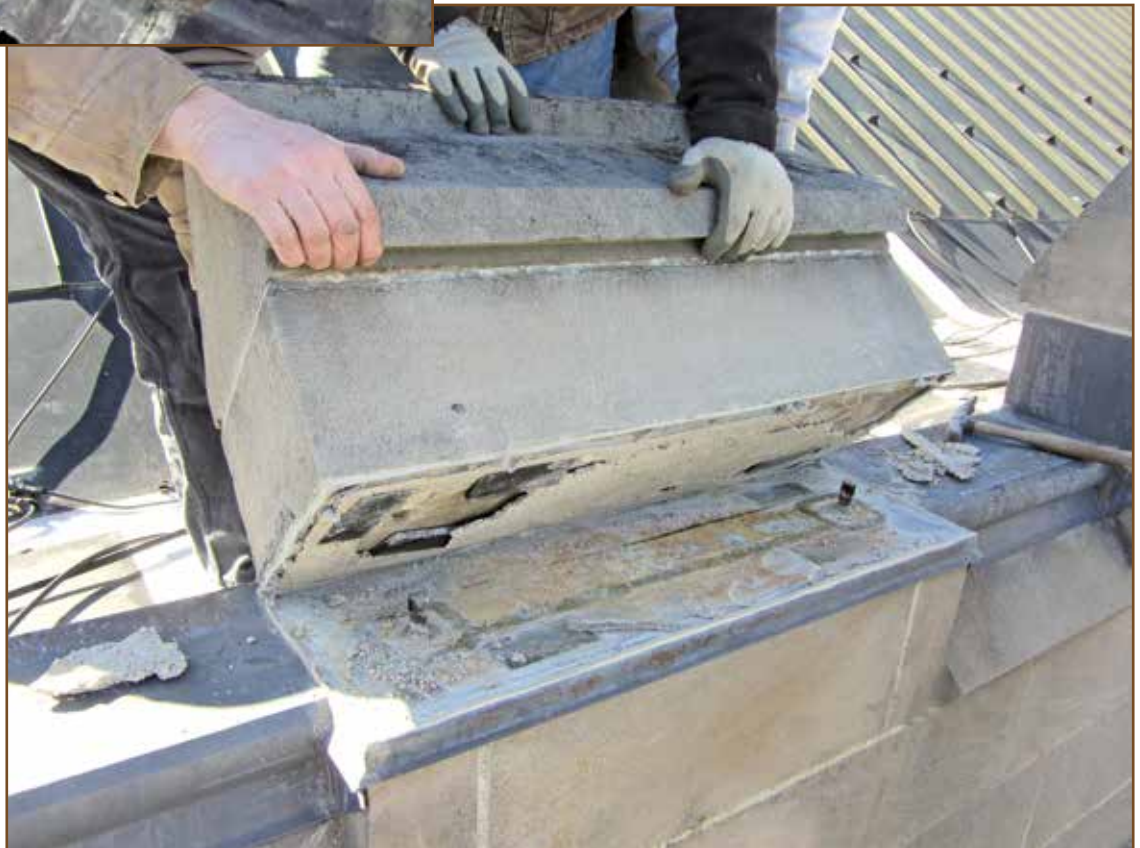
Photo 8 – Merlon stone attachment inspection (note 1-in. pin pipe).
