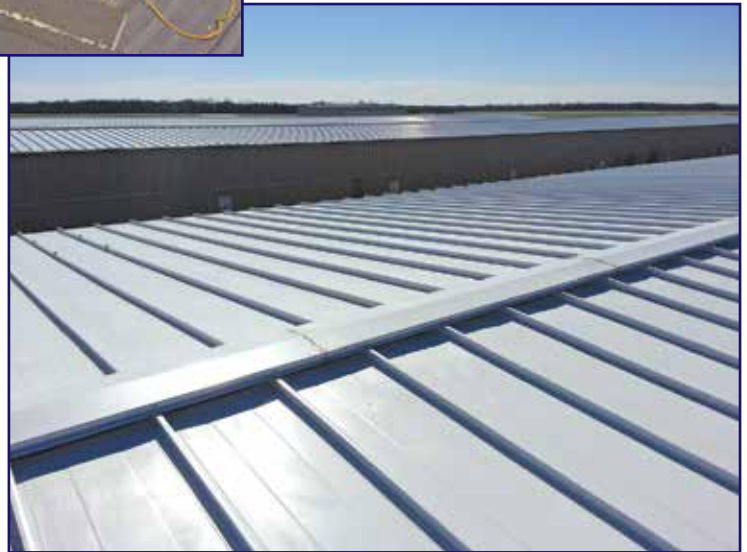
Figure 7 – A 24-in.-wide frameless symmetrical re-cover system with wind clamps in corner zone per FM requirements.
