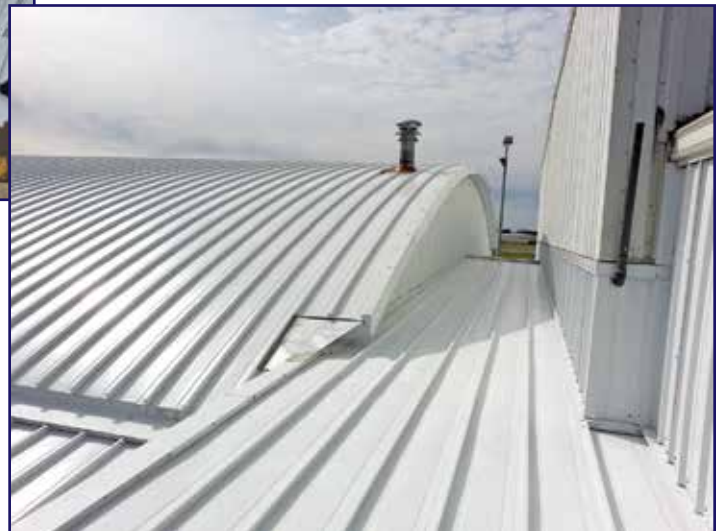
Figure 5 – Finished application showing continuous panel, step-down, and welded stainless flashing.
