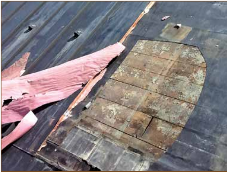
Photo 7 – 2000 EPDM underlayment assembly.
