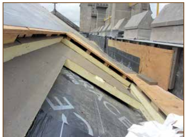
Photo 10 – 2012 vented and insulated roof assembly.
