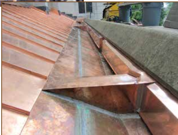
Photo 12 – Nave aisle roof gusset expansion joint and wall vent assembly (2012 installation).
