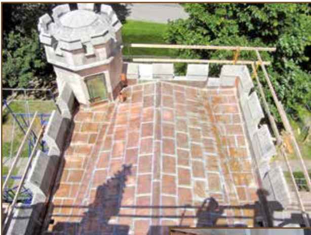
Photo 11 – 2012 semitranssept roof flat-seam copper installation.
