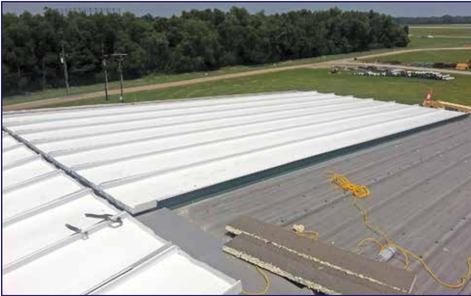
Figure 6 – Installation of the 24-gauge Galvalume symmetrical panels.
