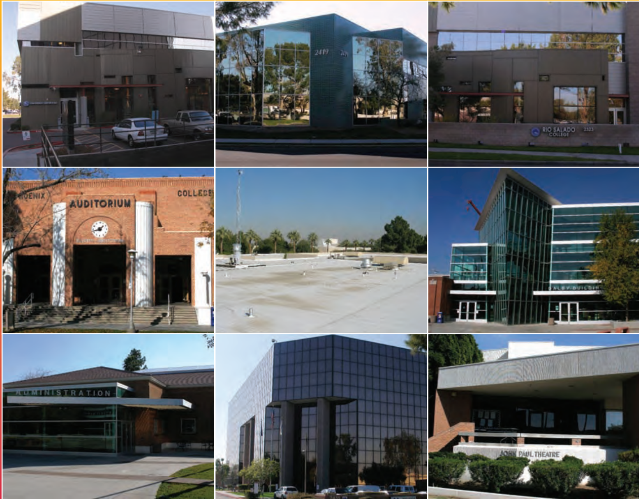
Photos courtesy of professional roofing consultant, WRECORP, Peoria, AZ
