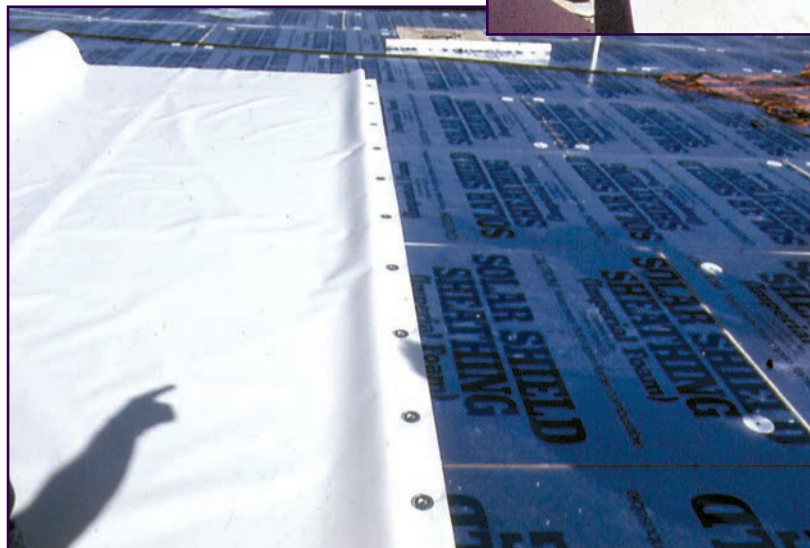
Figure 2: Factory-installed nailing tabs mean fewer seams to seal in the field..
