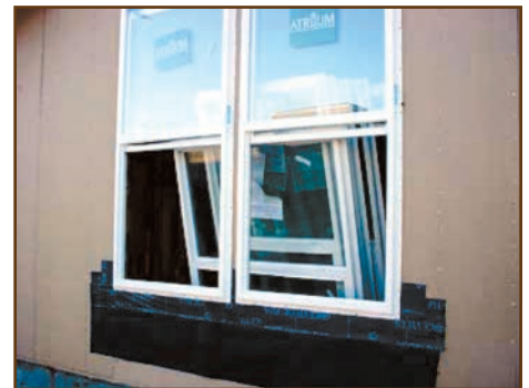
Figure 1: Examples of precut sections of building paper under windows to ensure proper lapping.
