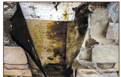
Figure 2: The consequences of reverse lapping.
