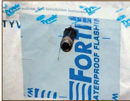
Figure 3: Penetration integrated into drainage plane.
