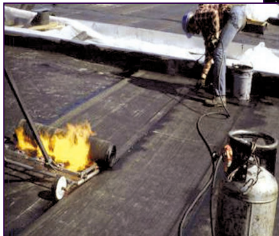
Figure 6: One layer of polyester mat laid in hot asphalt is a non-conventional single-ply roof membrane.
