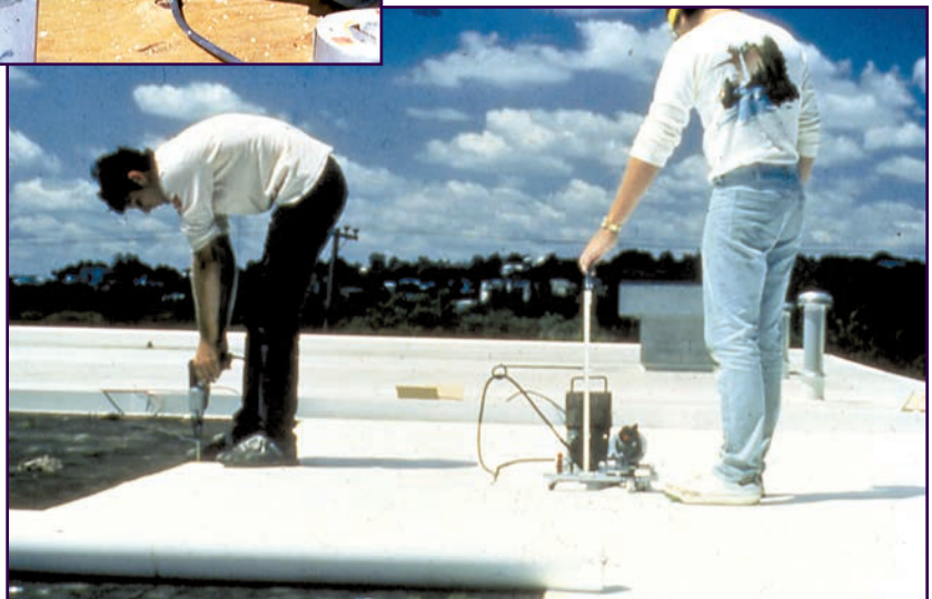
Figure 14: Lead weights have been stacked on this seam welder to improve CPE seam fusion.
