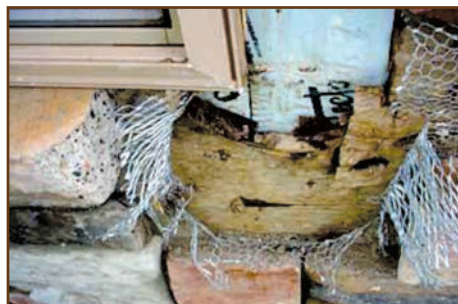
Figure 2: The consequences of reverse lapping.
