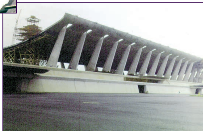
Figures 10A (left) and 10B (below): Dulles Airport required a flexible roof membrane to withstand expected structural movement.
