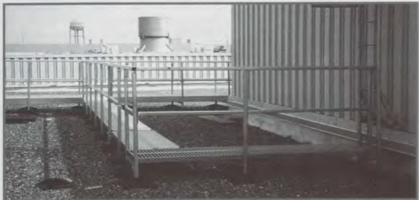
Pre-fabricated metal plank walkway system on built-up roof system.
