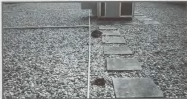
Concrete paver walkway for ballasted EPDM roof system.
