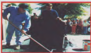
Michael Steele, left, and Randy Froelich, right of Siplast, Las Colinas, TX, demonstrated application of modified bitumen.
