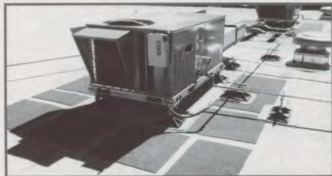
Modified bitumen walk pads around roof-top HVAC unit.
