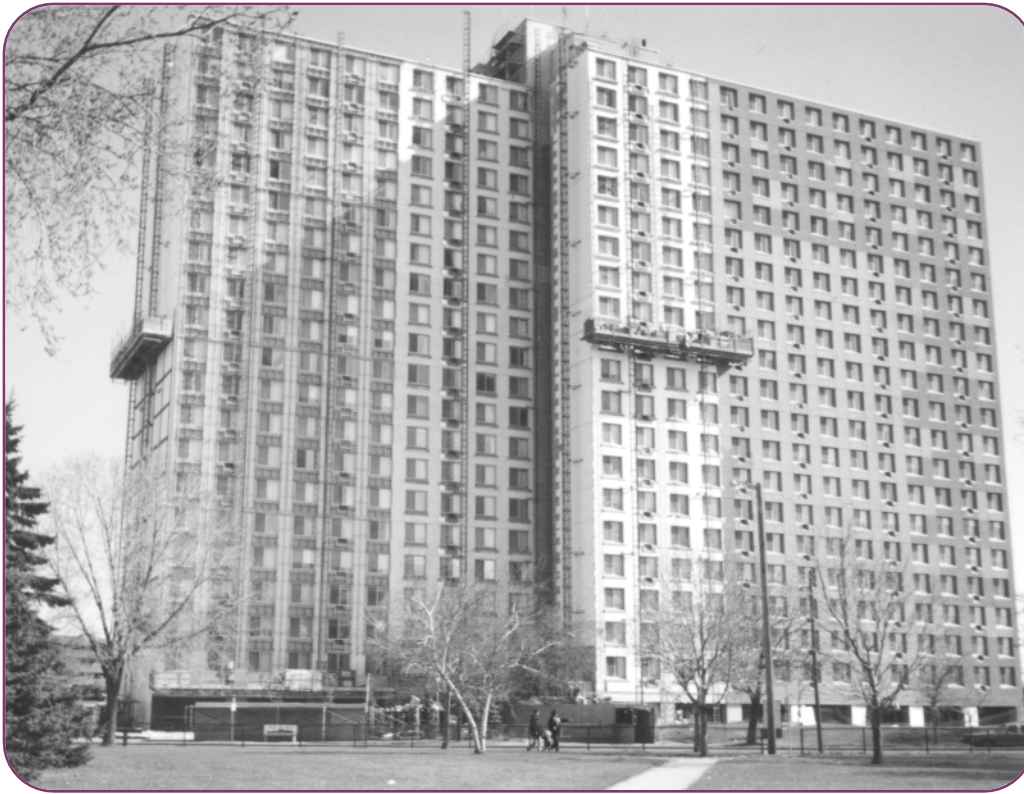
Figure 8—Elevation showing numerous windows.
