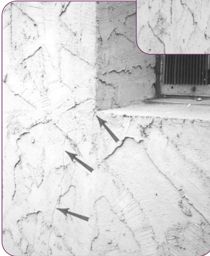
Above. Figure 1—Inadequate slope at original sill.
