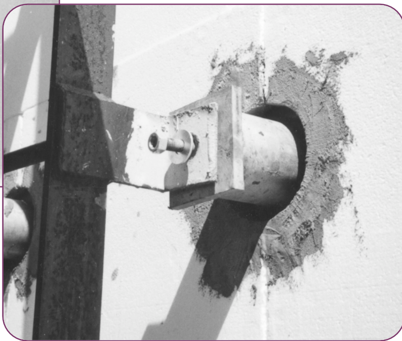
Figure 12—Stand-off ladder bracket.
