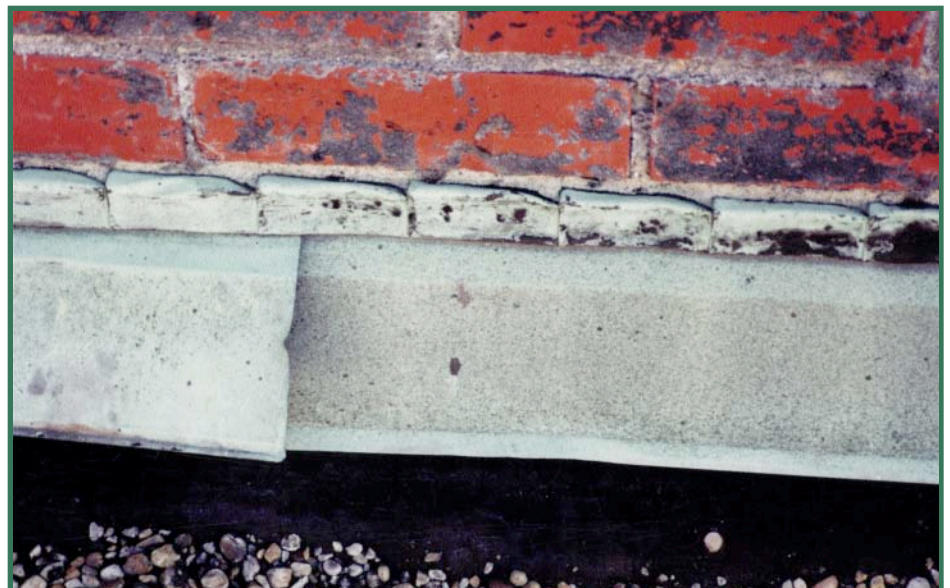
Figure 10—Historically, copper was the product of choice as flashing. The material is easy to form and joints can be closed with block tin solder.
