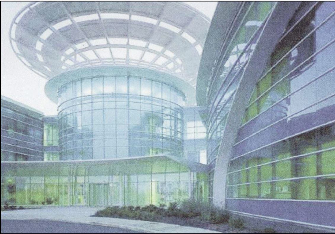
Figure 2—Applied Industrial Technologies, Cleveland, OH. Architect: GSI Architects, Cleveland, OH. Contractor: Turner Const. Co., Cleveland, OH. Glazing Contractor: Architectural Product Sales Co., Brooklyn, OH. Curtain Wall Framing: Vistawall CW-600 and W-250.
