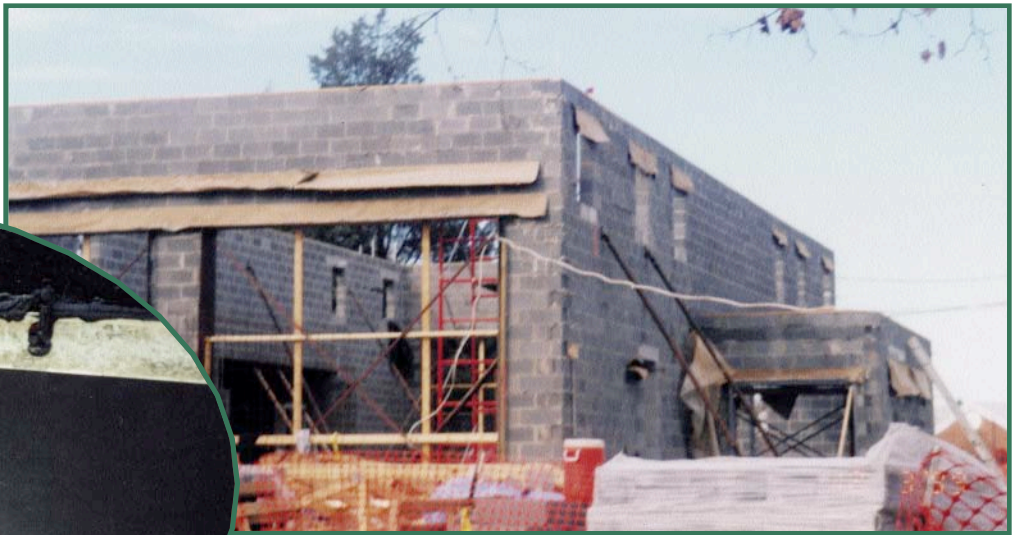
Figure 12—Asphalt-coated copper is now in wide use as the thru-wall flashing. It is easy to shape and can offer functional diversion of water when formed as a continuous component.
