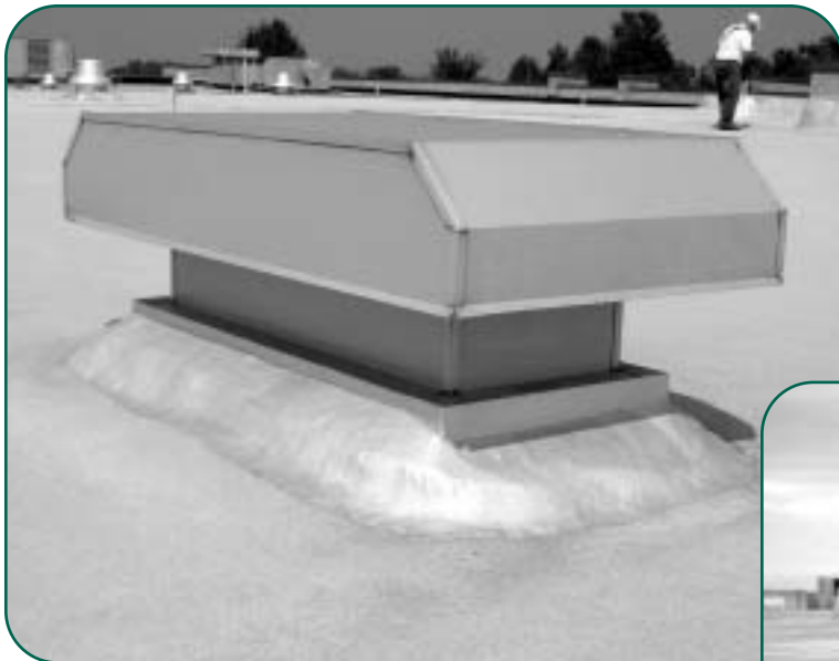
Figure 9 - Equipment support – high curb.
