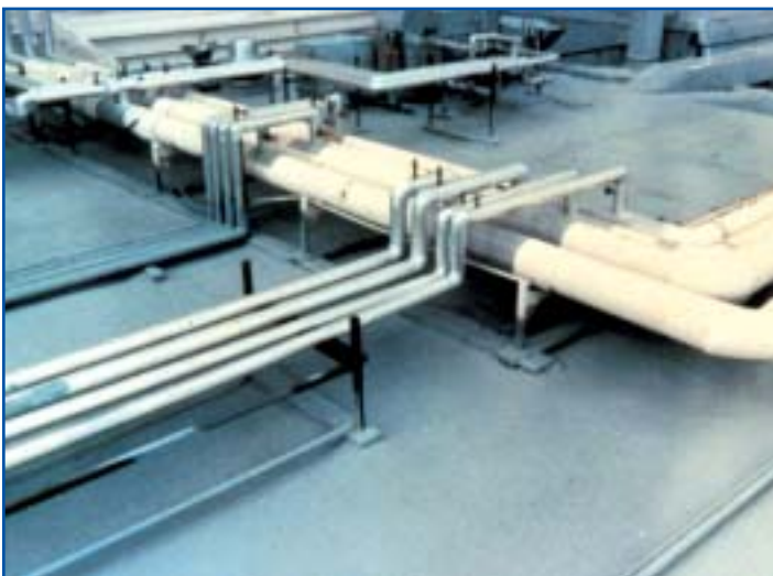
SPF is custom made for roofs with lots of penetrations.
