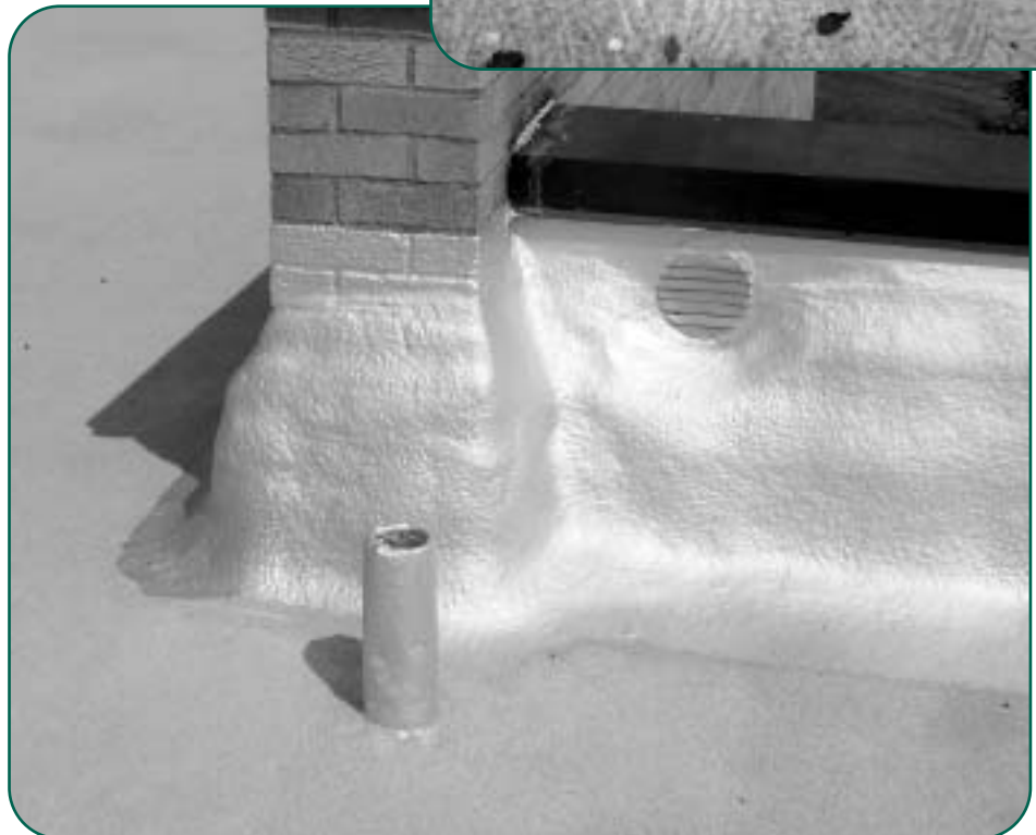
Figure 8 - SPF low wall flashing application.
