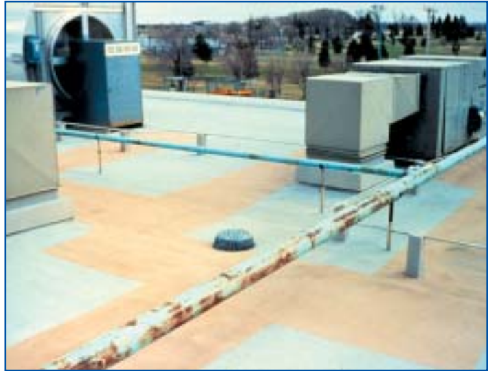
Roof mounted HVAC units should be raised and curbed, but typically don't require additional counterflashing.
