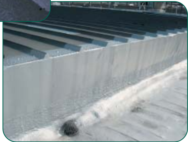
Figure 13 - SPF flashing, roof-to-wall.
