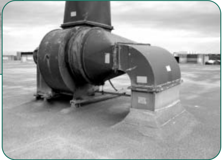
Figure 10 - Equipment support – low curb.
