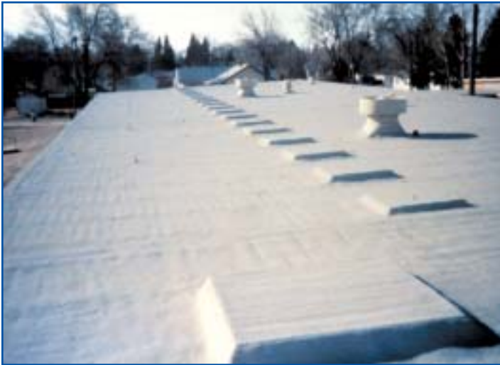
SPF helped to seal repairs made to this existing roof.
