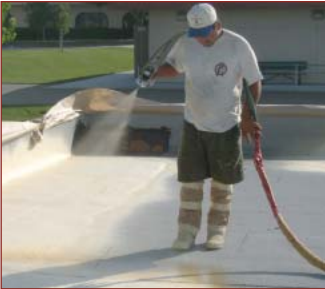
Application of SPF from trailer-mounted spray rig.
