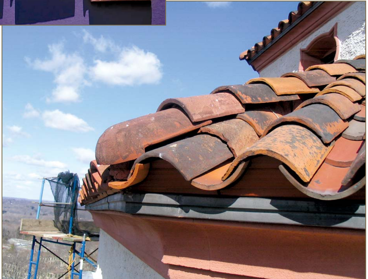
Photo 7 – Accessory tiles, such as the rounded hip closure tile shown above (or tiles for ridges, rakes, and starter courses) are often available from manufacturers for various tile shapes and styles. In some cases, these require special order and have considerably longer lead times than typical field tile shapes. Identify and order accessory or custom tile shapes early to avoid delays during construction.
