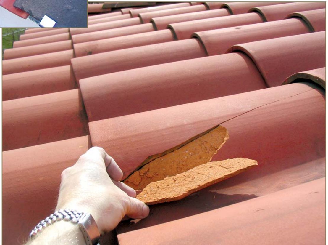
Photo 4 – Delamination in clay tile as a result of freeze-thaw damage. Testing of clay tiles prior to selection and installation can help avoid such damage.
