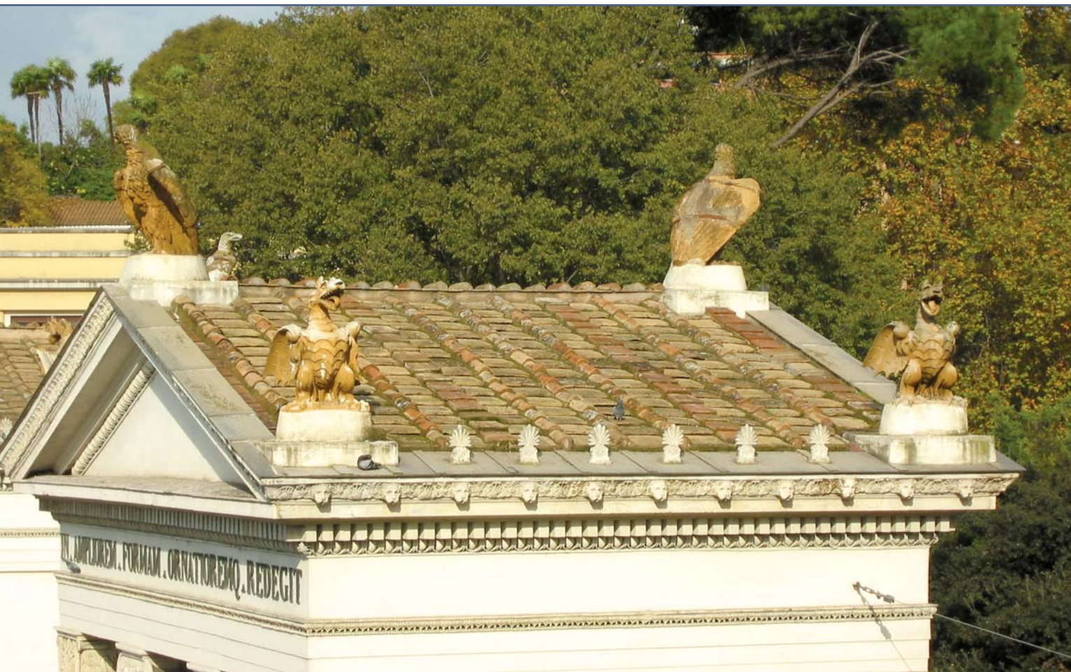
Photo 2 – Flat clay tile in the Piazza del Popolo, Rome, Italy. Photo courtesy of Robert L. Fulmer.
