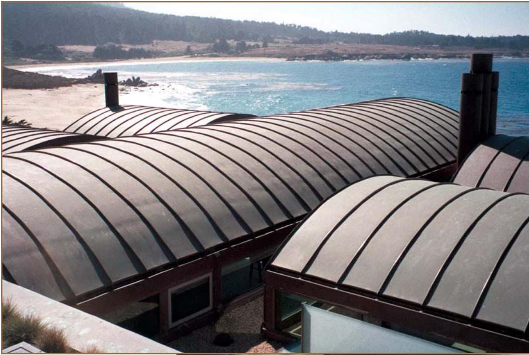
Photos 5 (left) and 6 (below) – Saturated plywood sheathing below self-adhering membrane underlayment in a non-vented barrel roof with a standing seam copper covering.
