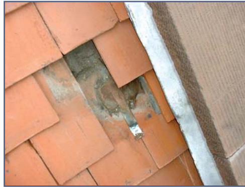
Photo 4 – Clay overlapping (flat shingle) tile exhibiting signs of water absorption. Photo by Robert L. Fulmer.
