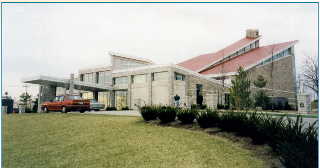
Figure 1: General view of the roof.
