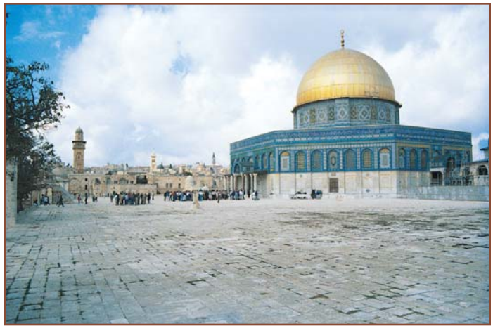
The Dome of the Rock, finished in 691 following the Turkish conquest of Jerusalem, is believed to have originally sported a gold roof. It is now gold leafed aluminum. (All photos courtesy of Metal Roof Advisory Group, Ltd.)
