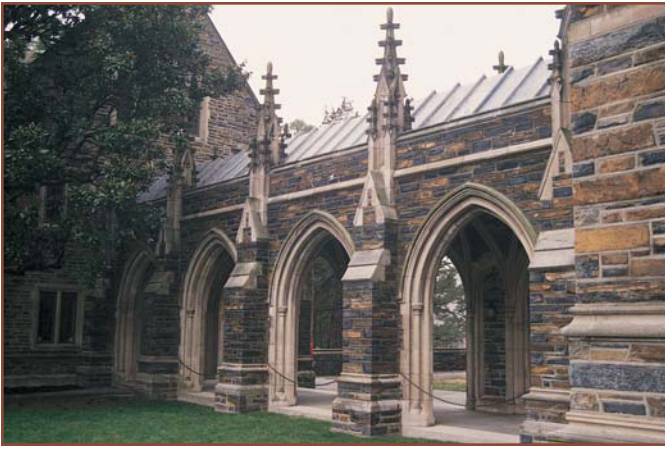
This LCC batten roll roof on the Chapel of Duke University (above) was installed in the late 1930s. The craft of metal roofing was brought to North America by such European artisans as Paul Revere.
