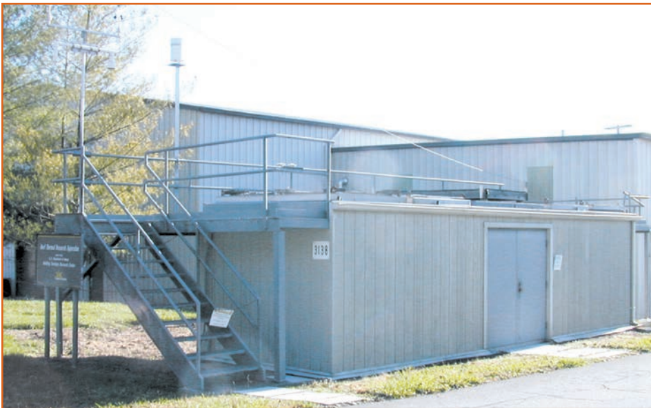
Figure 1: Roof Thermal Research Apparatus (RTRA) with weather station.
