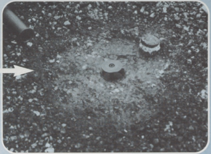
Fastener in place ready for pullout.
