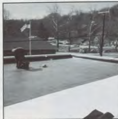
The new roof has two membranes: one black and one white.
