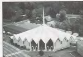
St. Malachi's Church Eterna-Seal over Urethane Foam
