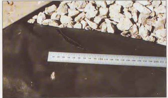
Fig.: 2 Close up of existing expansion joint.
