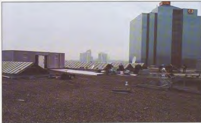
Fig. 10: The completed roof with roof expansion joint installed.
