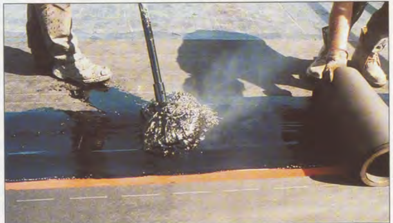
(Left): Fig. 6: The roof expansion joint being installed in a flood coat of asphalt.
