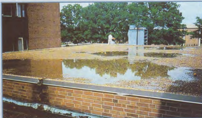
Overview Roof Area B.
