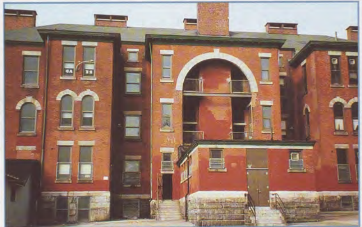
Overview, rear of Edwin H. Fitler Elementary School.
