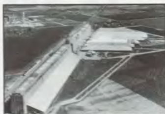
Garvey Grain Co. Eterna-Seal over Metal
