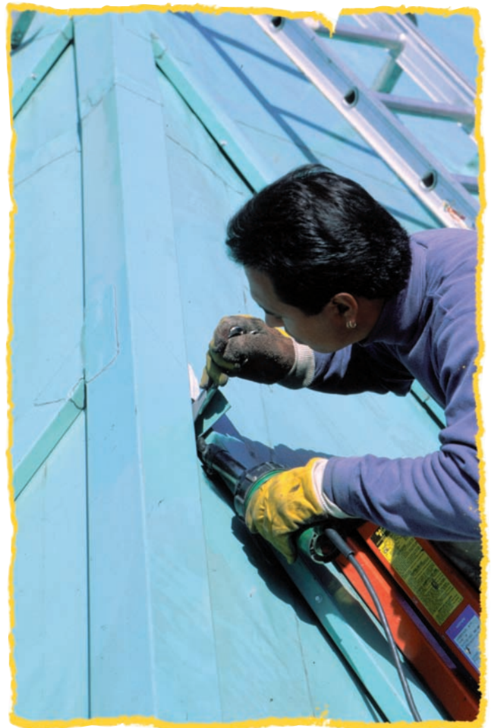
A workman performs hot-air welding on a joint detail.
