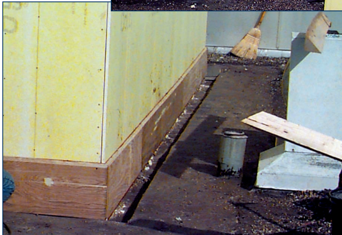
Below: Revised proper flashing conditions with required wood blocking.
