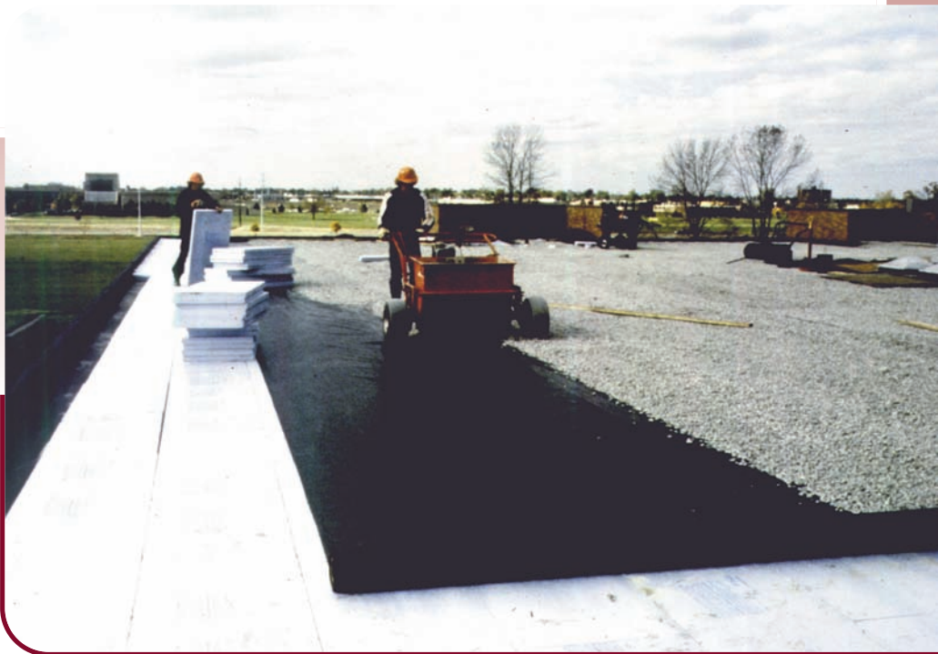
Figure I—Typical PMR system being installed.
