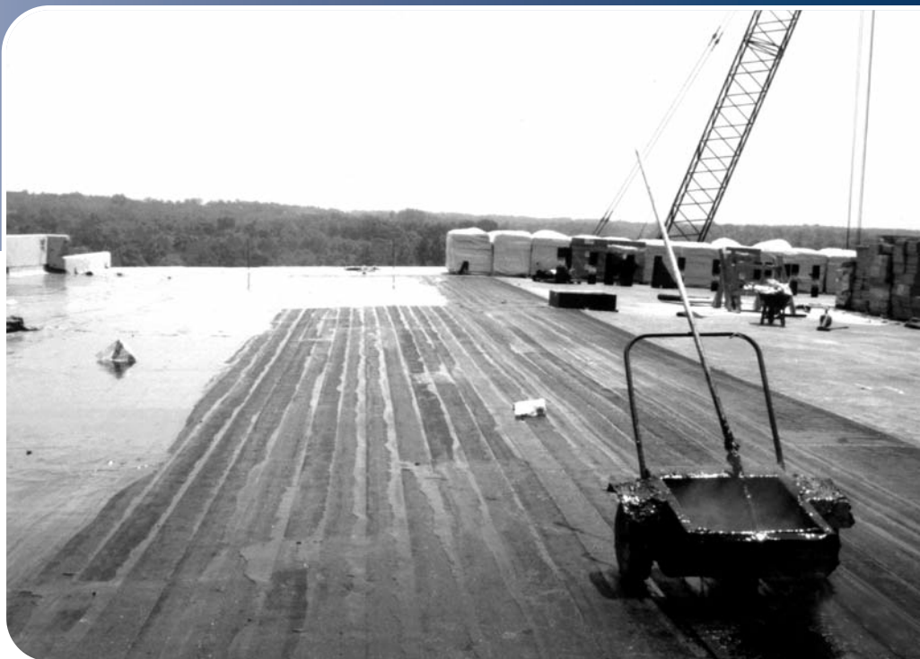
Figure IV—BUR membrane on concrete deck.
