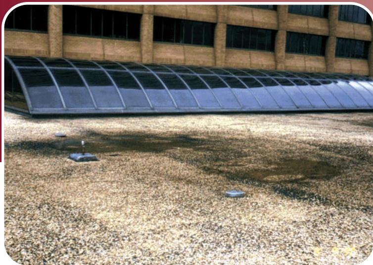
Figure VII—Picture of Connector Roof on Sloppy Floyd Building.
