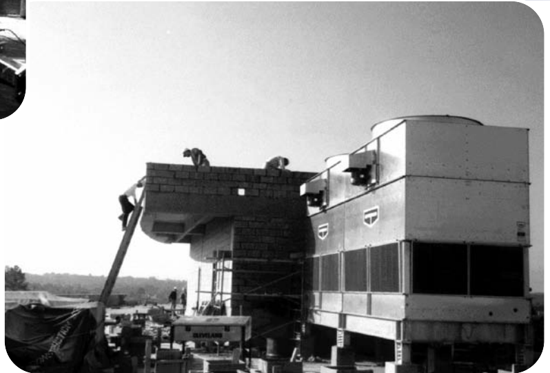
Right: Figure VI—Trades working on Royal Center III.
