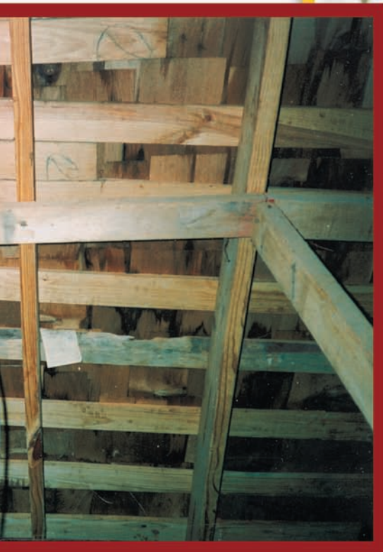
Left: Figure 4—Spaced support sheathing is a preferred arrangement for wood roofing products (although this carpentry is marginal). Observing daylight from below a wood roof covering on spaced strapping does not always signal substandard construction.
