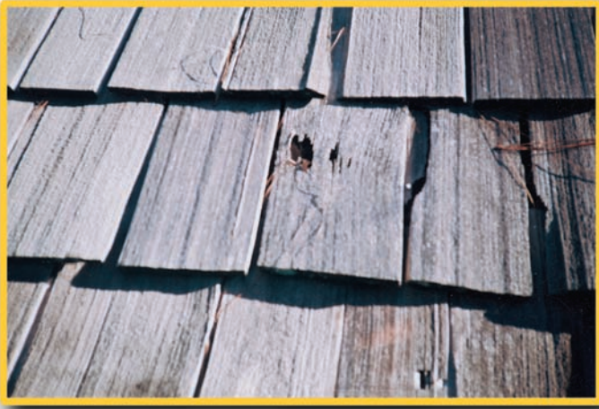
Figure 7—Some installers are unqualified or unwilling to cull unacceptable materials. This shake has a significant knothole and should not have been used.
