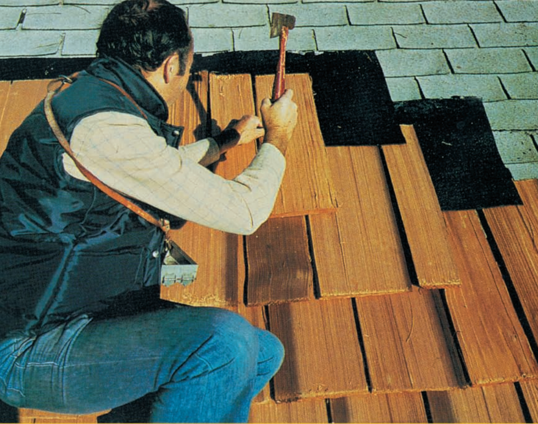
Above: Figure 3 —Over-roofing with shakes may inhibit the underside air circulation so vital for wood roofing products. However, over-roofing can be accomplished in a functional configuration.
