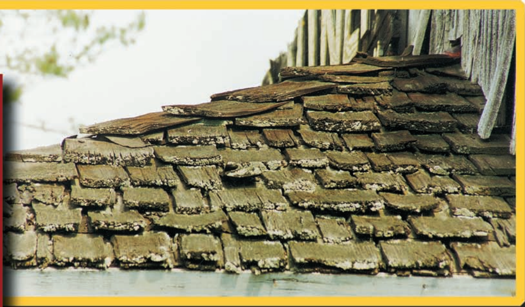
Left: Figure 4—Spaced support sheathing is a preferred arrangement for wood roofing products (although this carpentry is marginal). Observing daylight from below a wood roof covering on spaced strapping does not always signal substandard construction.
