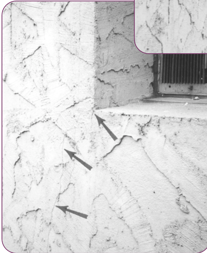
Above. Figure 1—Inadequate slope at original sill.
