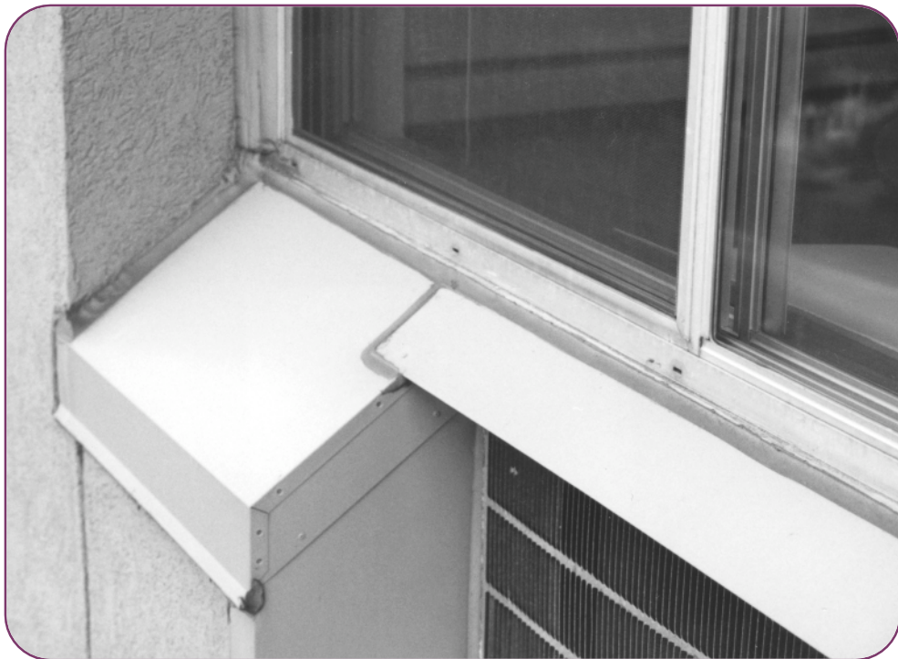
Figure 7—Sill and A/C opening with new sheet metal flashing.
