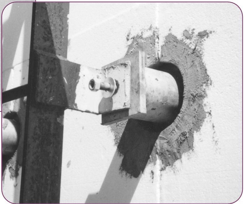
Figure 12—Stand-off ladder bracket.
