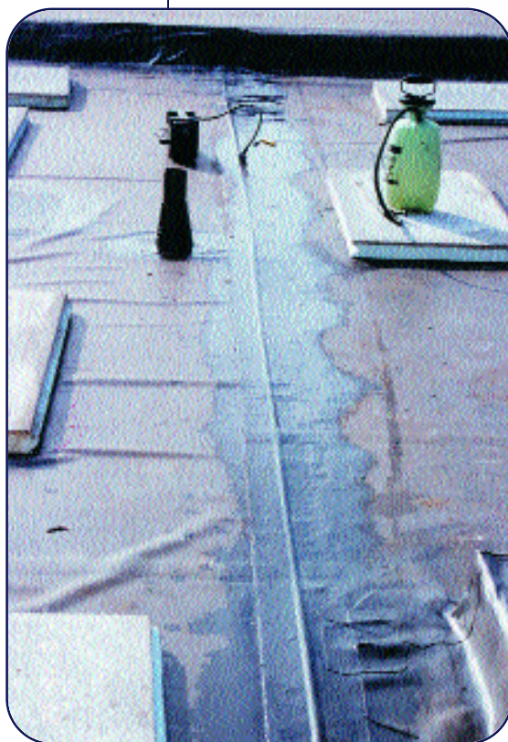
Above: Exhibit 3: Application of seam cover with bond breaker at center line develops a void to accommodate pressurizing the opening in order to test continuity and quality of seam bond.
