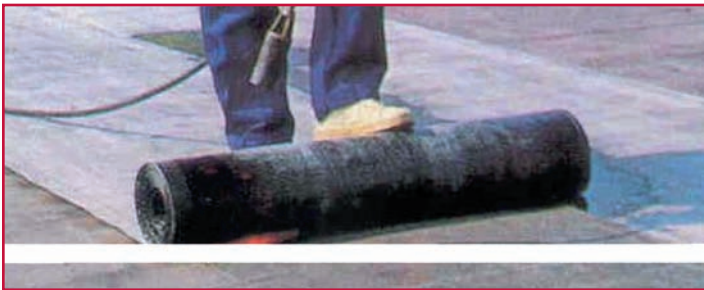
Photo 9—There is a greater potential for blistering when the torch is applied directly to the Dens-Deck® surface.
