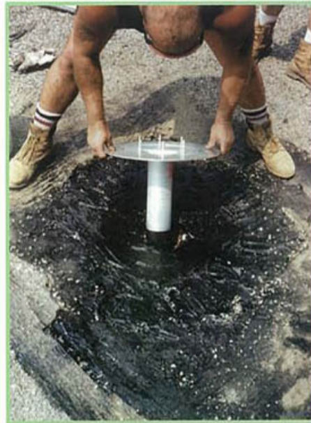
Retrofit drain being inserted into original drain bowl by roofing contractor.
