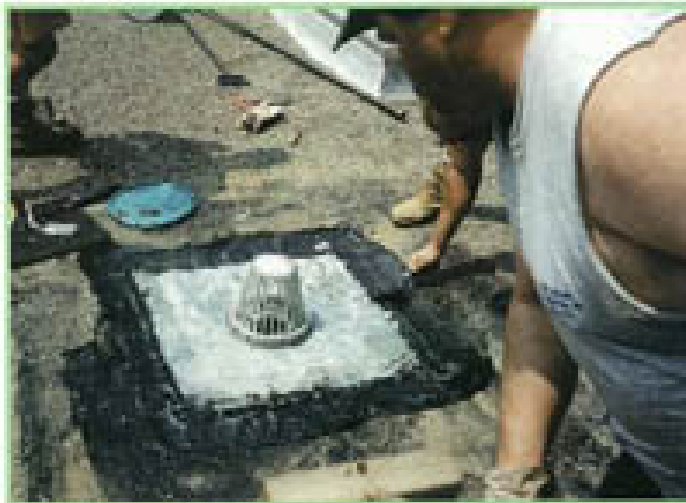
Roofing contractor putting finishing touches on retrofit drain flashing.
