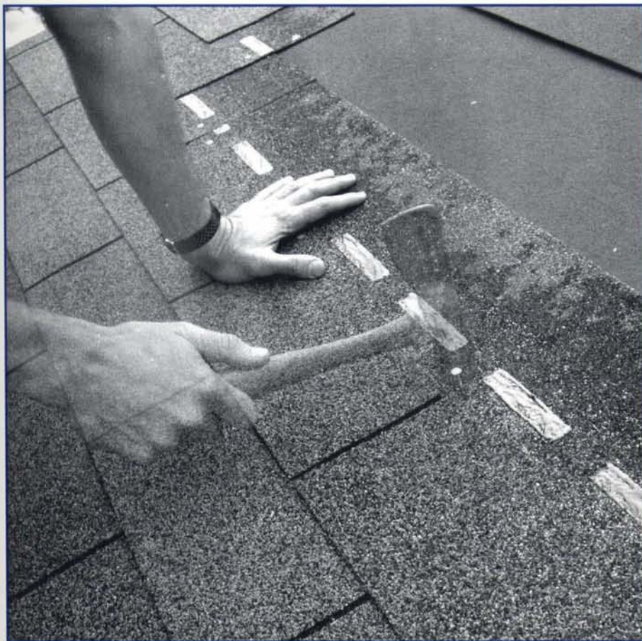
Application of SBS shingles.
