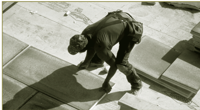
A worker installs board insulation.
