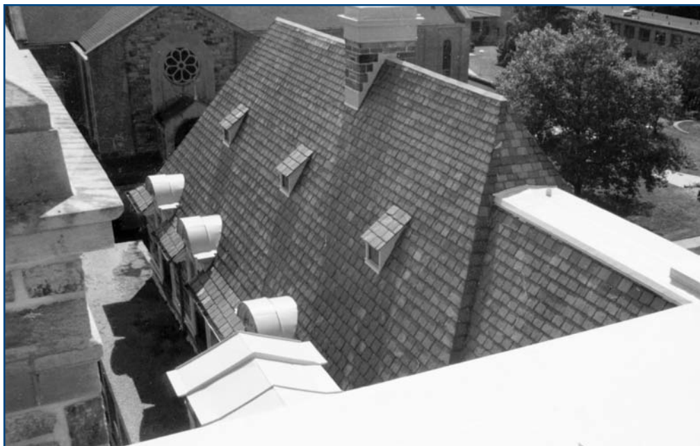
Pigmentation options are limited, but thermoplastic elastomers are well suited for pastel applications such as this patina green at the Aldrich mansion in Warwick, Rhode Island. (Photo courtesy Roof Work Inc.)
