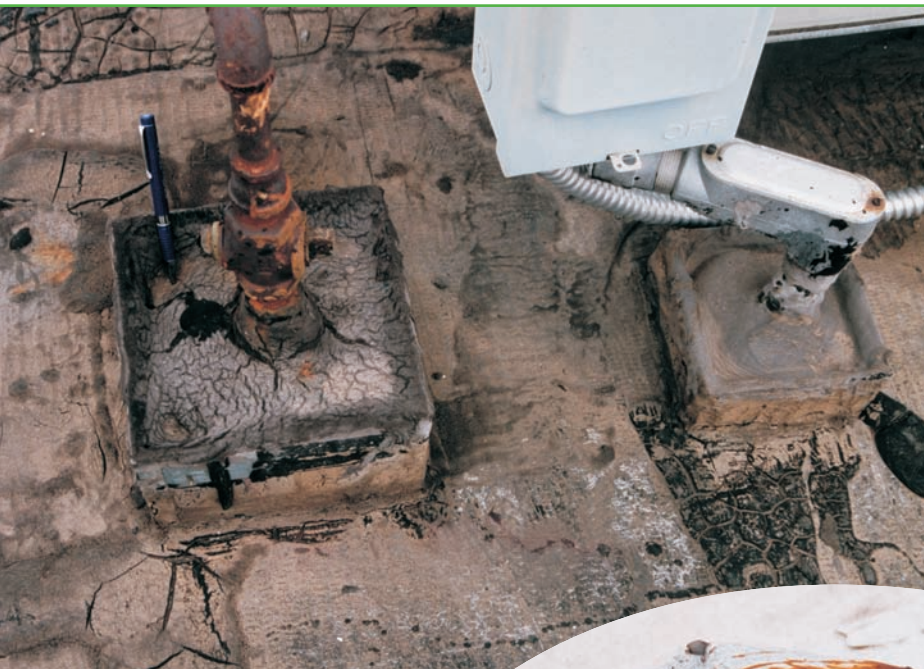
Above: NRCA pitch pans on a built-up roof.
