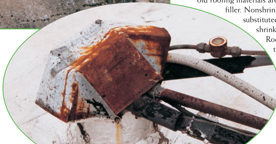
Above: NRCA pitch pans on a built-up roof.
