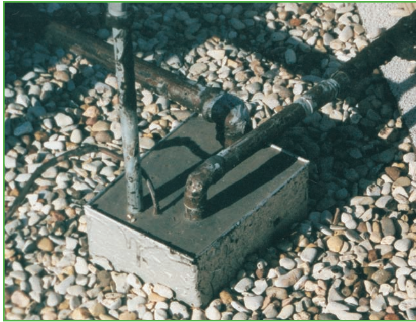
SPRI-approved pitch pan on EPDM.
