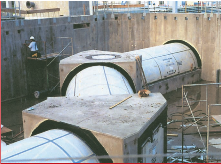
Figure 9 – One of the large marine tanks at Newport Aquarium during construction.
