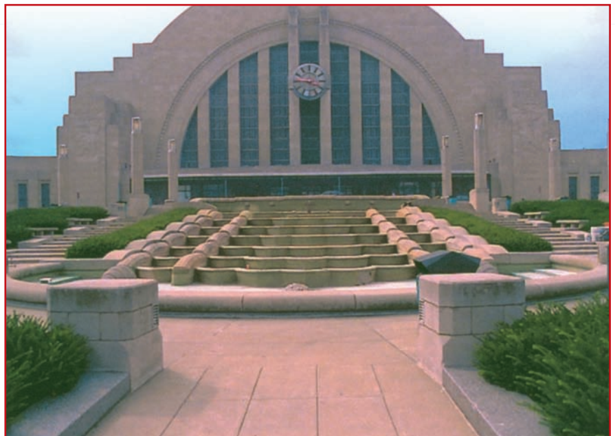
Photo 1 – Overall view of the Cincinnati Museum plaza fountain
