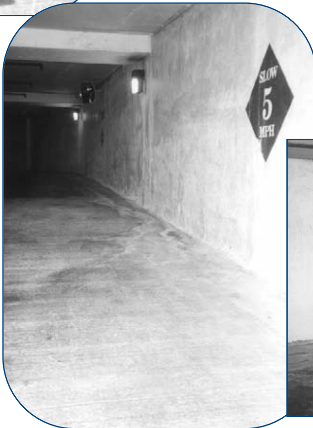
Figure 6: Above, left, epoxy injection sealed the leaking construction joint shown in Figure 4 against static pressure of the surrounding water table. Figure 7, above, right: Wet, treacherous areas around the base of the ventilation shaft shown in Figure 5 are dry after epoxy injection of wall cracks, although leaks were continuously active, and cracks were contaminated with bentonite. (Photos by Phil Haisley.)
