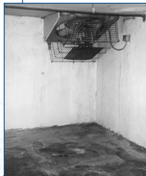
Figure 6: Above, left, epoxy injection sealed the leaking construction joint shown in Figure 4 against static pressure of the surrounding water table. Figure 7, above, right: Wet, treacherous areas around the base of the ventilation shaft shown in Figure 5 are dry after epoxy injection of wall cracks, although leaks were continuously active, and cracks were contaminated with bentonite. (Photos by Phil Haisley.)
