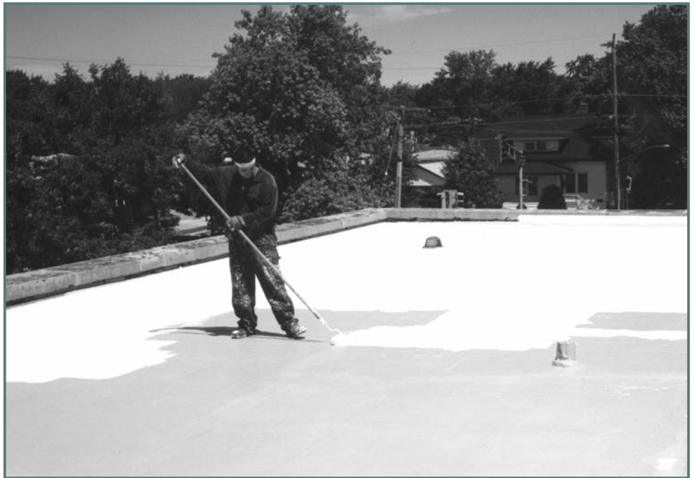
Photo 2. The installation of reflective membranes or coatings meeting the EPA's Energy Star® Roof Products Program has the potential to reduce urban heat gain as well as pollution by lowering air conditioning loads. Meets Tenet 13.
