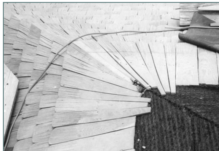
Photograph 9—Completed fanned hip construction.
