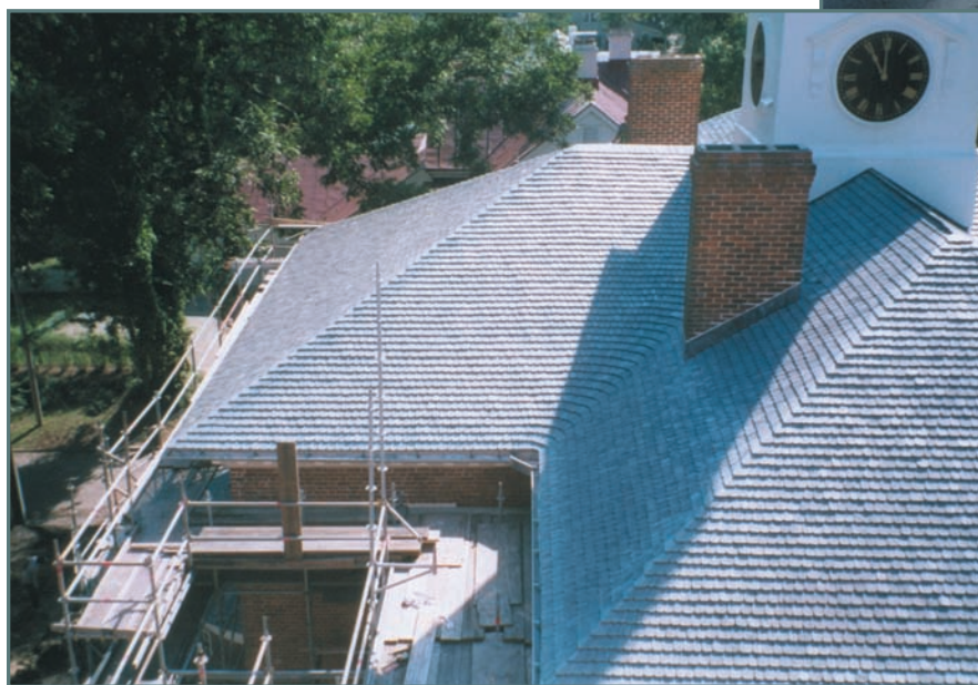
Photograph 2—New cypress shingle roof.
