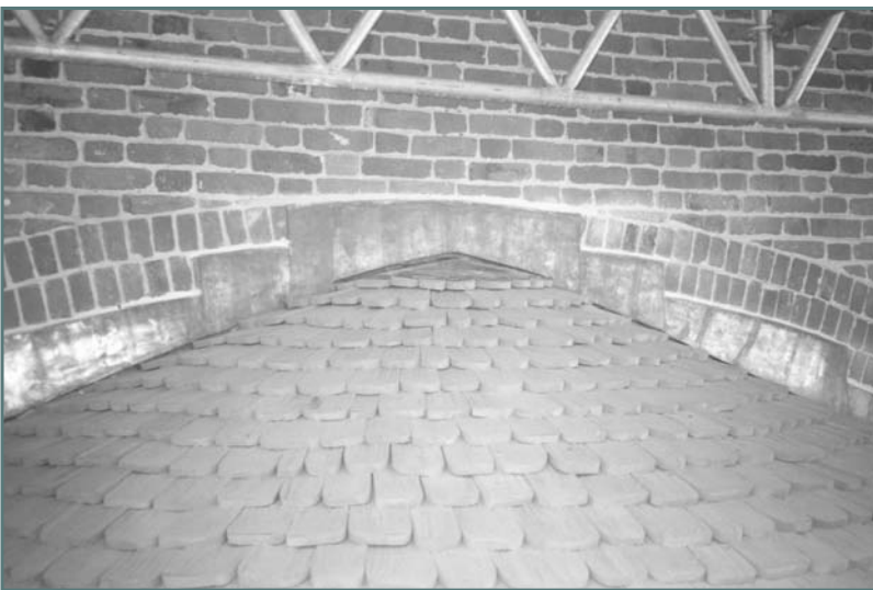
Photograph 12—Fanned shingle installation at apse.
