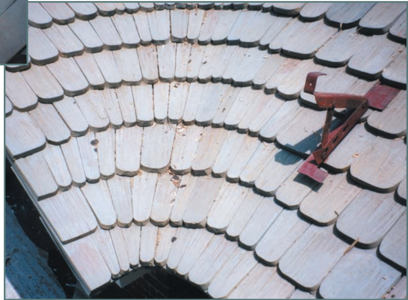
Photograph 6—View of completed swept valley.
