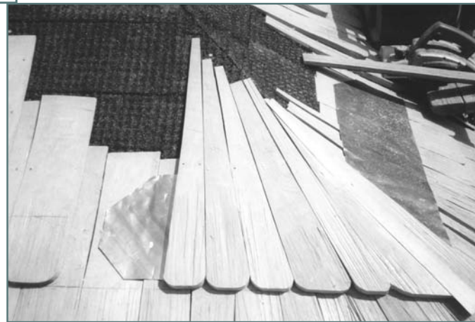
Photograph 8—Fanned hip construction. Shingle to right side of hip has been mitered and lapped; however, the butt remains to be trimmed.
