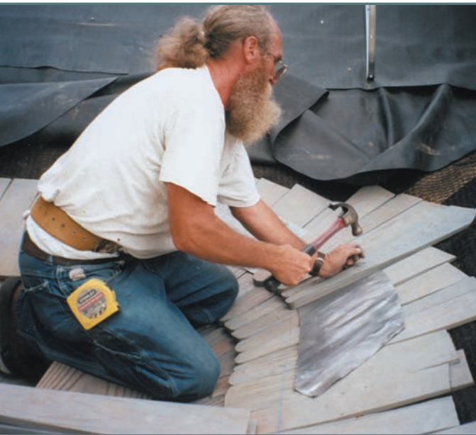
Photograph 5—Buddy Tate constructing a valley. Note the 18" shingles approaching the valley, the 24" shingles within the swept portion of the valley, and the lead flashing.
