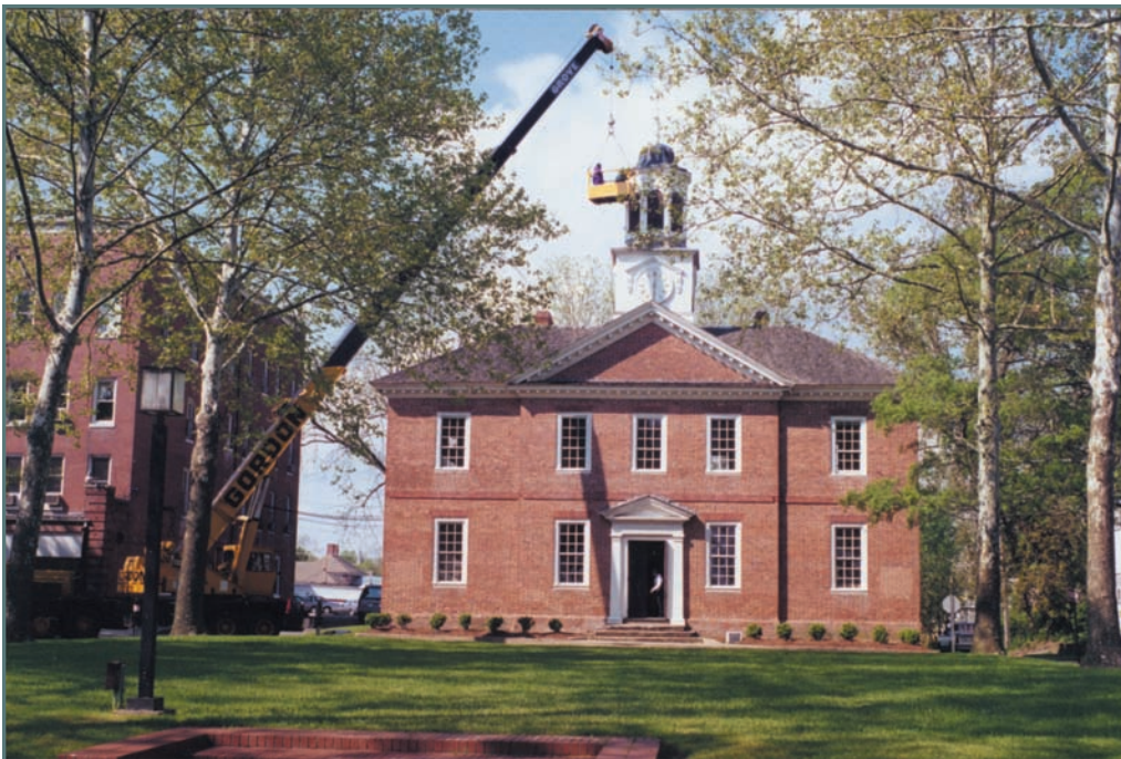
Photograph 1—Before renovation. Roof investigation in progress.
