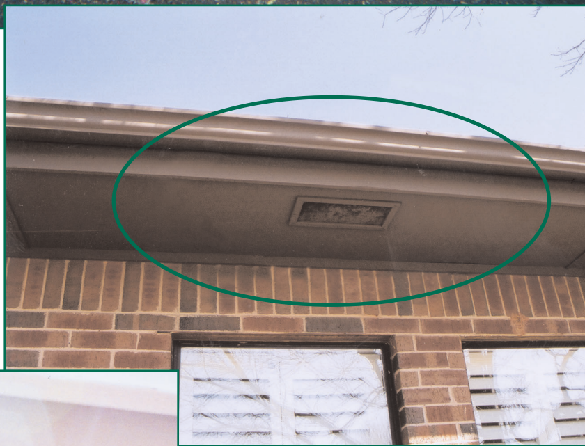
Figures 5a and 5b—Multiple coats of paint can render soffit openings virtually useless. Airways and vent openings should be slightly larger than would be implied in the sizing calculation.
